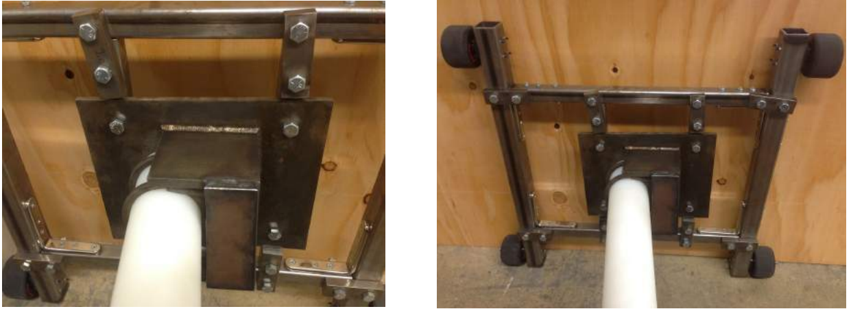
Figure 15.7. Pole Attachment In Enclosure on Platform
