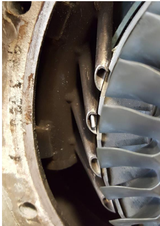
Figure 62. Stage 3 thermocouple inserted through the air-start rakes
