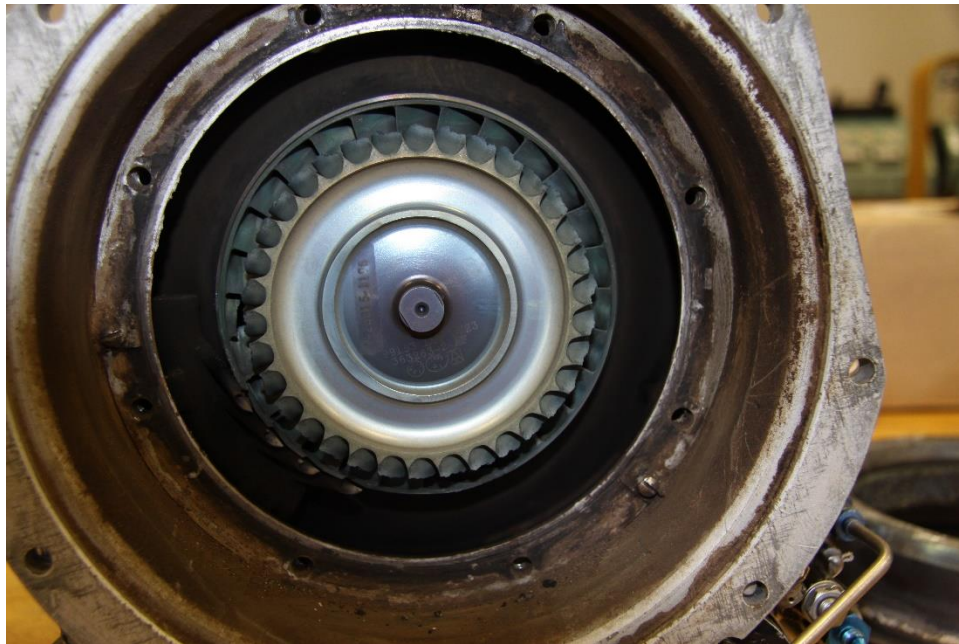
Figure 7. Gas-generator turbine blades after over-temperature condition
