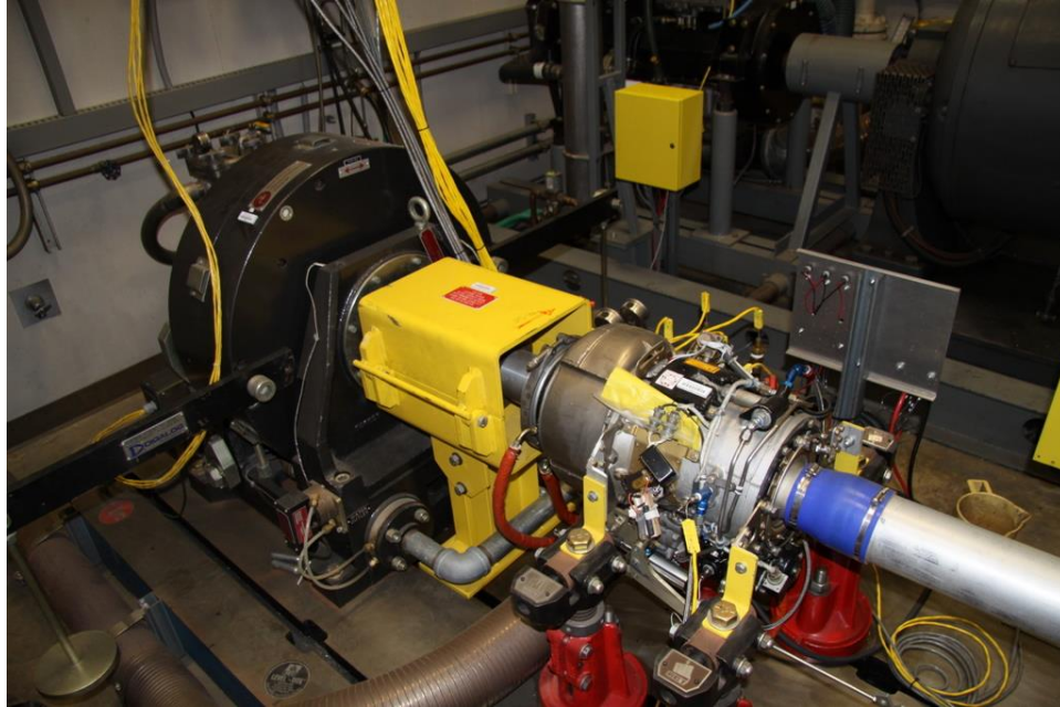
Figure 4. Completed installation of the JFS in the test cell.
