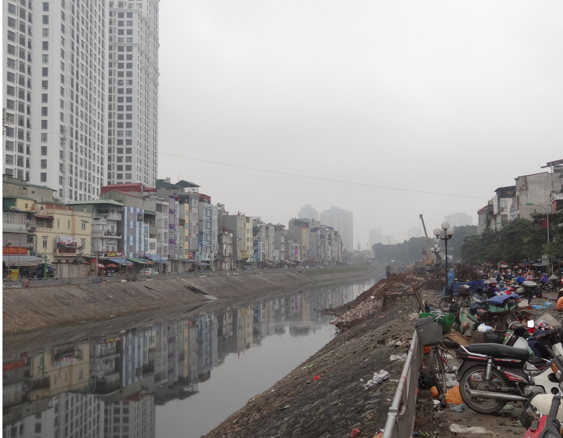
Photo: To Lich River, Hanoi's main drainage channel (©S. Fuhrmann, 2014)
