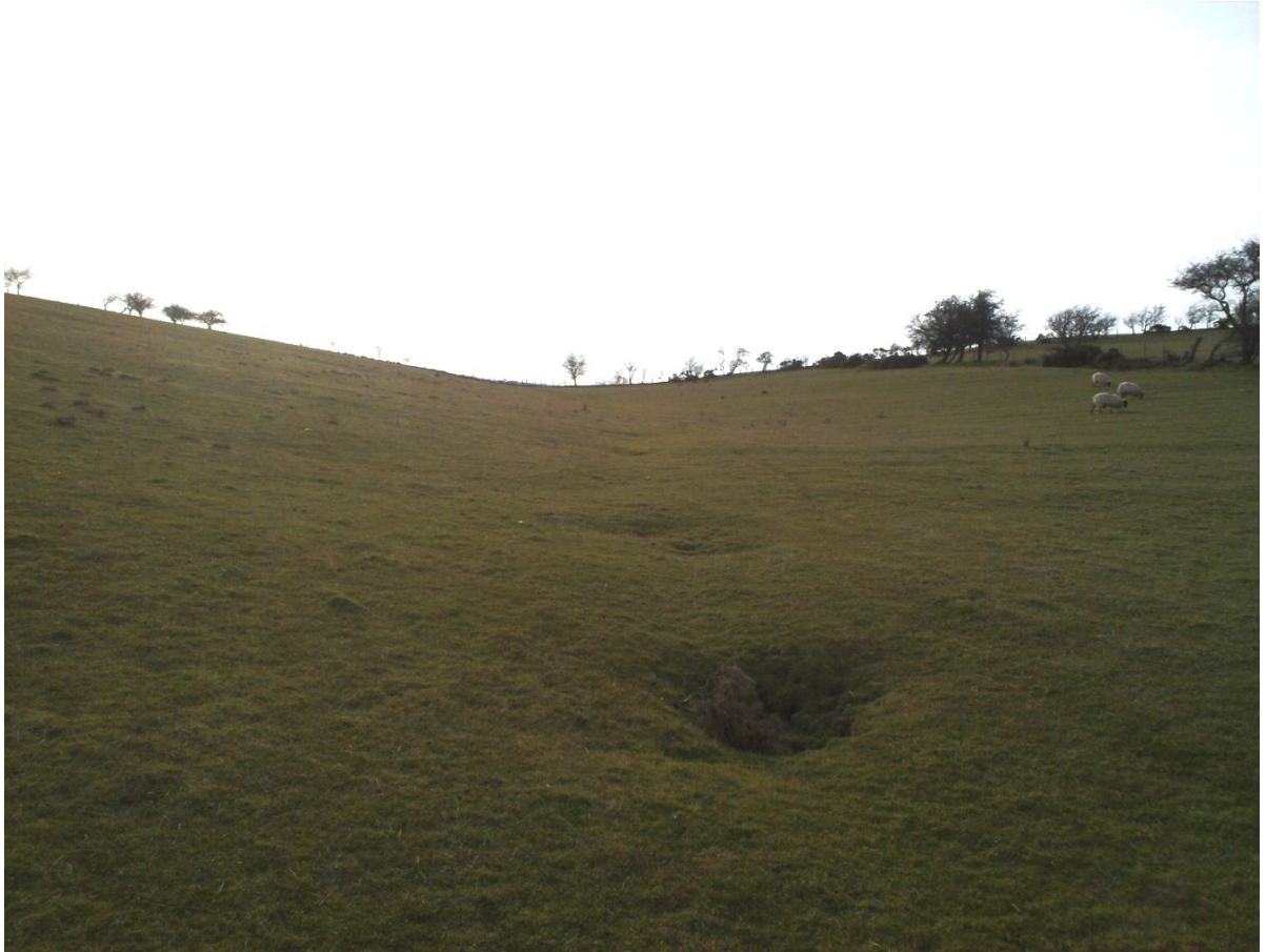
Figure 3.5: View upstream of the channel from the sump showing drain excavations as a result of the broken drainage pipe.
