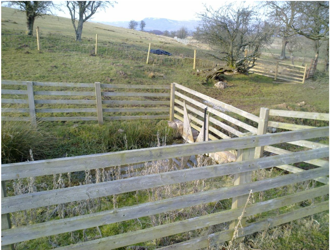
Figure 3.6: Image of V notch weir and sump.
