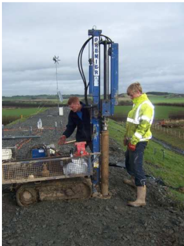
Figure 7.15 – Cutting of the borehole.
