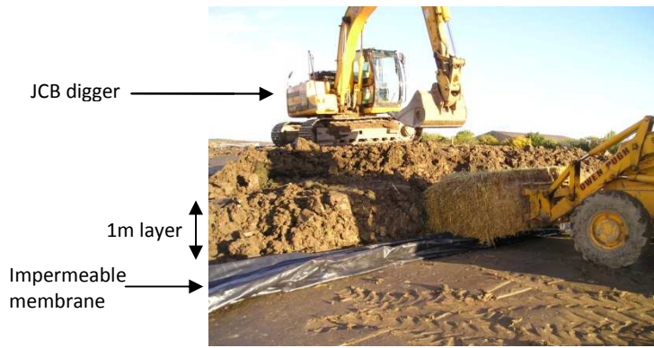
Figure 3.3 – Construction of a poorly compacted panel using a JCB, (Hughes, 2005).
