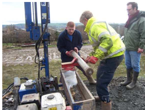
Figure 7.16 – Recovering the core of the borehole.
