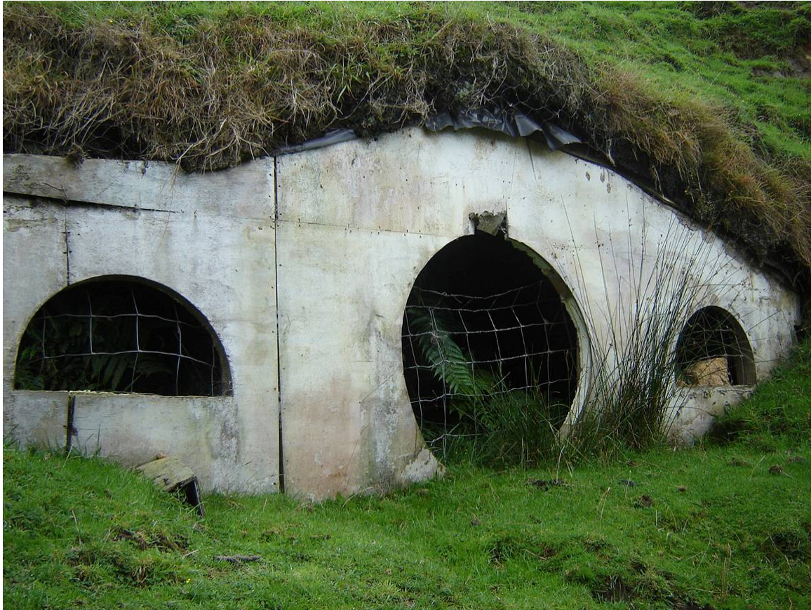
Image 70- A hobbit hole slipping into desuetude- for now. After some struggle, the Alexander family have been allowed to undertake repair work on the facades. This hobbit hole was awaiting renovation at the time of our visit.
