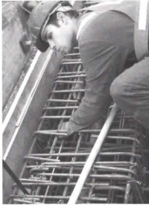
Figure 8: SOFO Sensor Being Installed in a Concrete Bridge Deck
