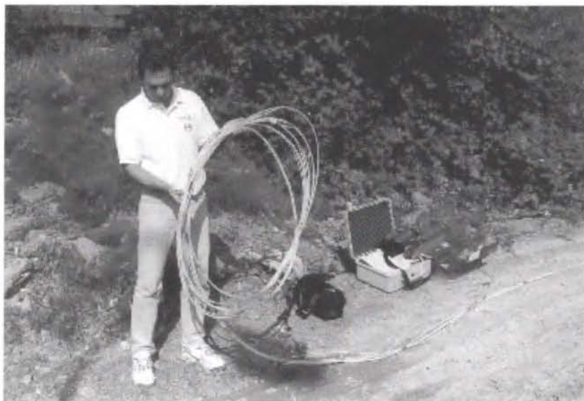
Figure 9: Bundle of SOFO Sensors Ready for Installation in a Pile for Lateral Friction Analysis
