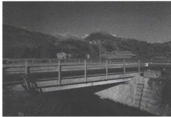
Figure 20: The bridge in November 2004, after rehabilitation and widening.
