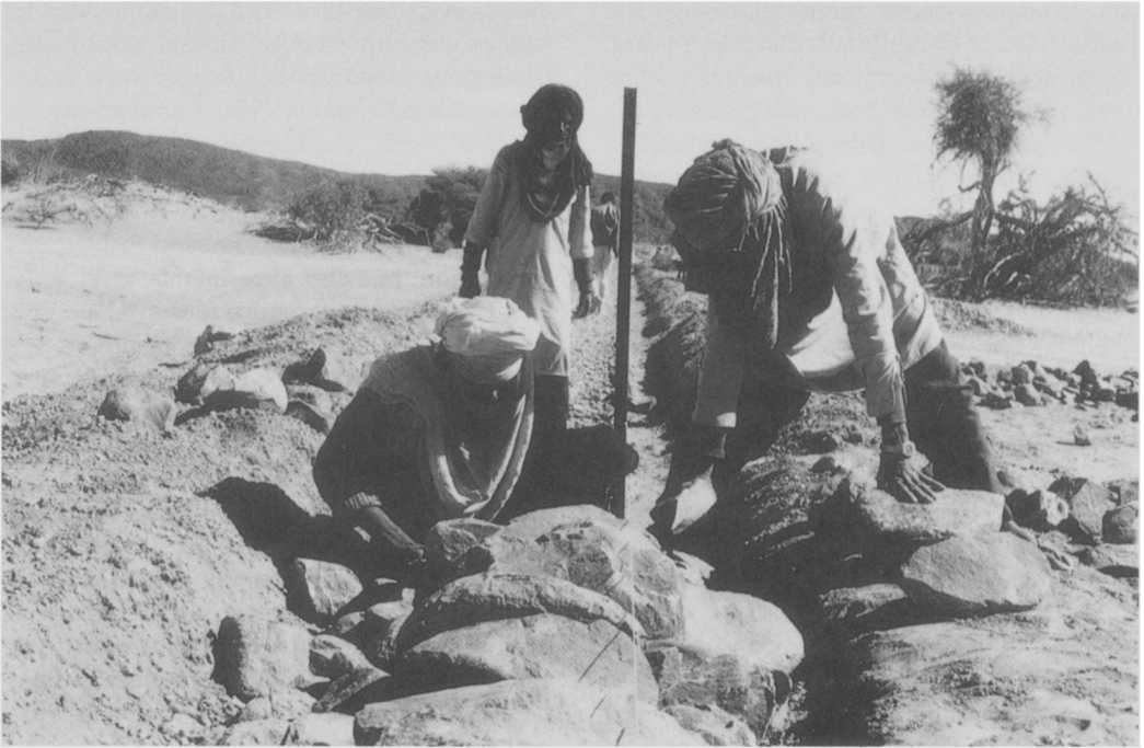
Appropriate technology and local materials allow local people to manage their environment in a sustainable way. Here a low, drystone dyke is helping reclaim degraded land ( Meg Gawler/WWF ).
