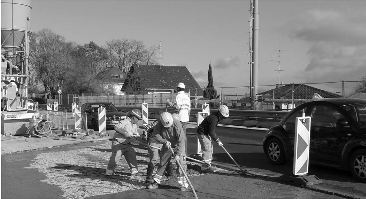
Figure 6: Underpass “Creux de Genthod” – nearby Geneva (CH), 2010, rehabilitation of a bridge deck with SH-UHPFRC, slope 5 %, average external temperature 5 °C
