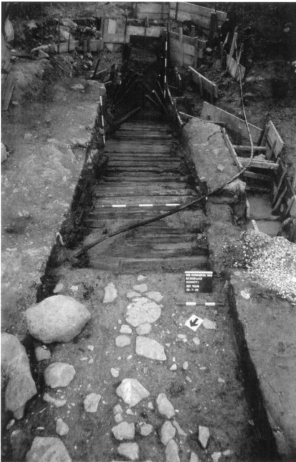
Fig 13. Dürrnberg-Sportplatz: the entrance or Mundloch running north-south with fully preserved timbering. In the foreground is the small entrance hut and an access way paved with pebbles. Towards the rear, the timbering of the adit uses the Mann-am-Mann technique, with cross-beams at top and bottom as well as side supports fixed by mortice-and-tenon joints. Photograph: T Stöllner
