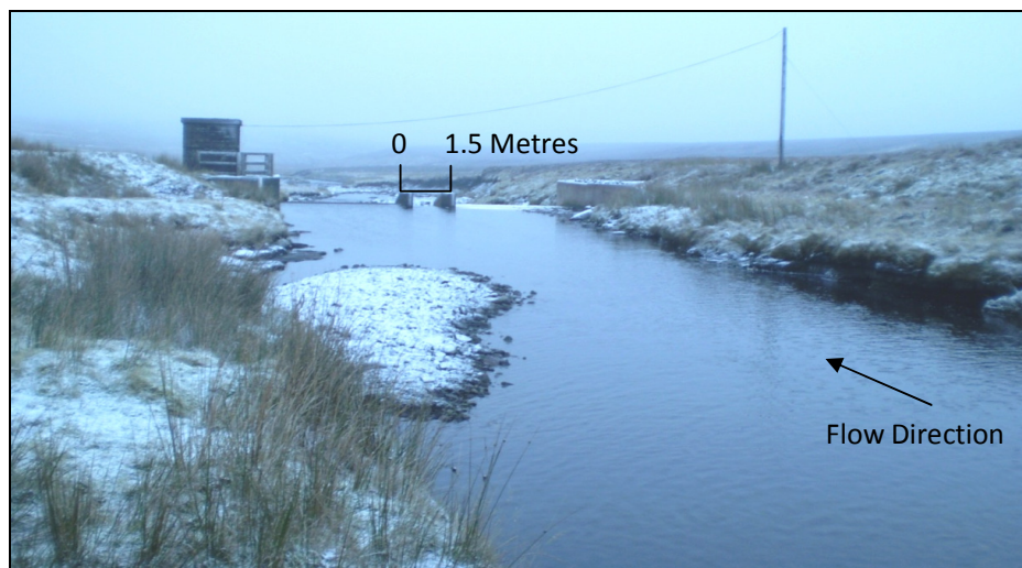
Figure 3.1 EA compound weir gauging station on Trout Beck, downstream of the study reach.
