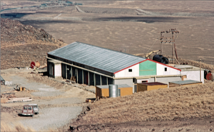
PLATE 2 — The US satellite tracking station under construction in 1968.
