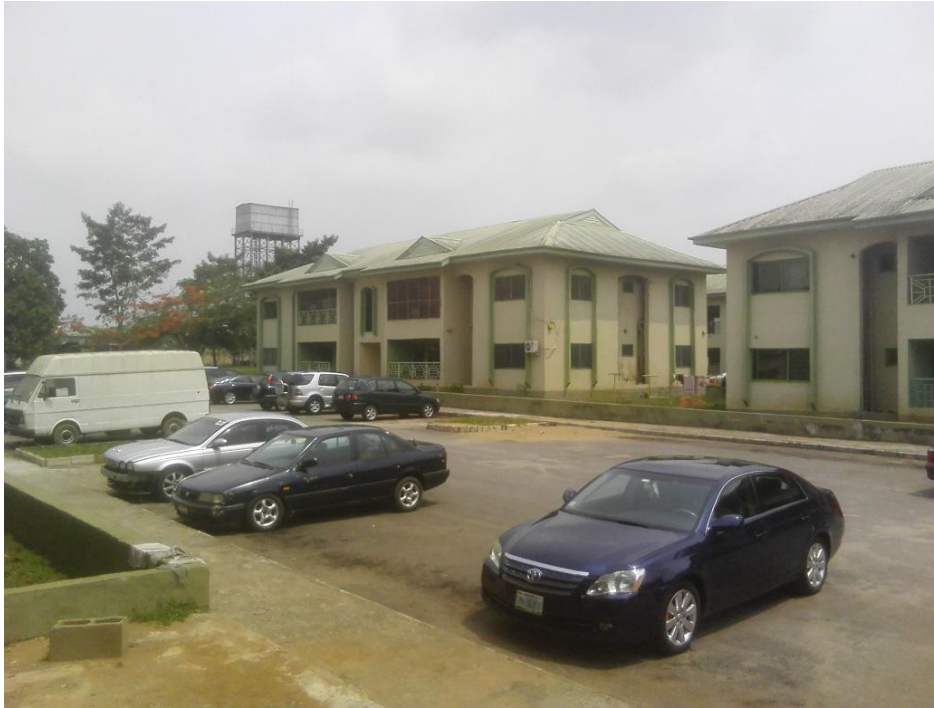
Fig. 3 A view of some residential quarters which is serviced by one elevated tank (shown in the background)
