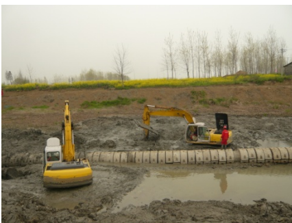
Figure 6: Adding heavy stuff onto gas pipelines
