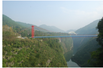
Figure 7: Picture of Yesanhe cross-cliff river pipeline-bridge
