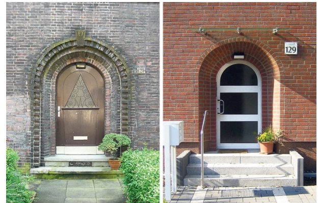
Figure 10. Energetic redevelopment of a housing estate in Dortmund, Germany. Entrance of Kronprinzenstraße 129 before and after. The left side shows unpretentious ornaments and patina on the facade. On the right side the former charm is covered under insulation packaging and brick imitation.
