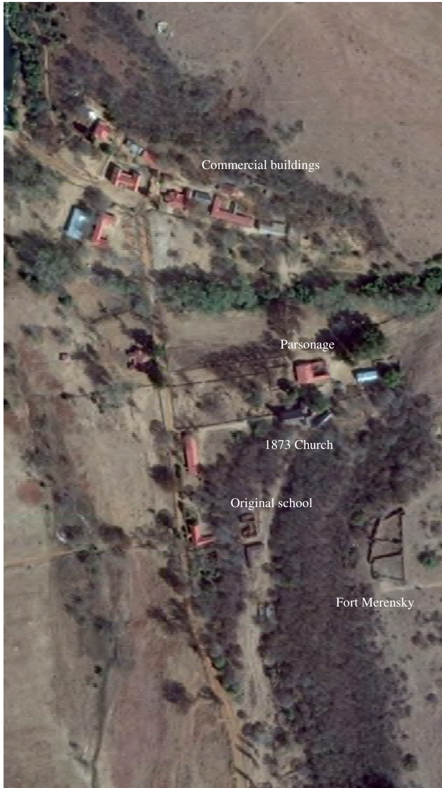
Figure 3.3: An aerial view of the Botshabelo Mission Station complex.
