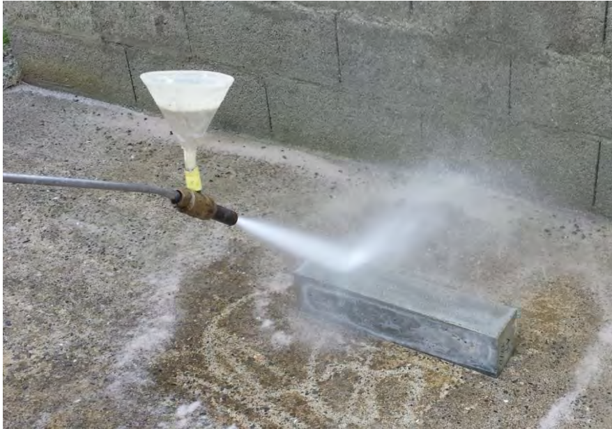
Figure III-2: Substrate surface prepared by sandblasting
