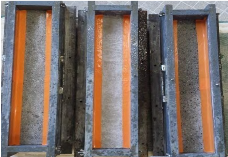
Figure III-7: Notch created by adhesive tape before casting repair
