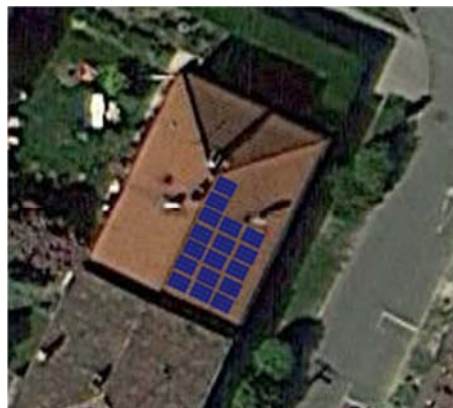
Fig. 6. PV modules allocation
