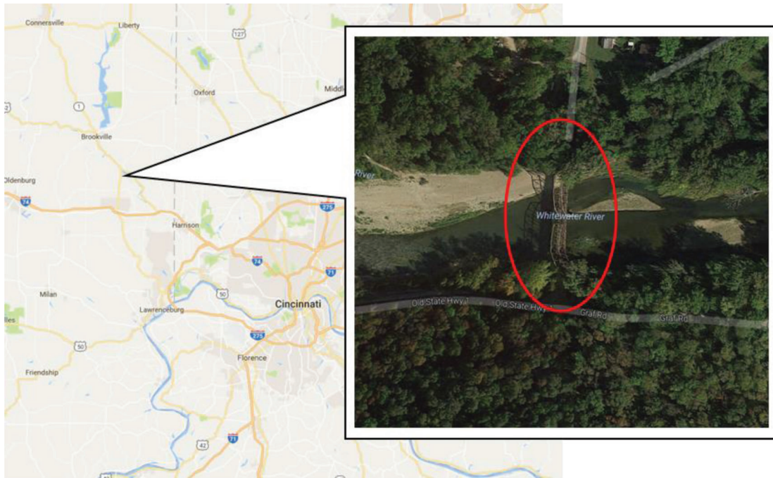
(a) Old State Road 1 Bridge over the Whitewater River in Cedar Grove
