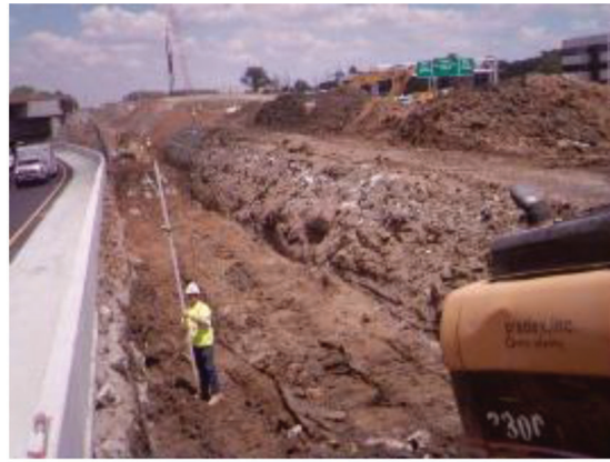
(b) Check level for pad
