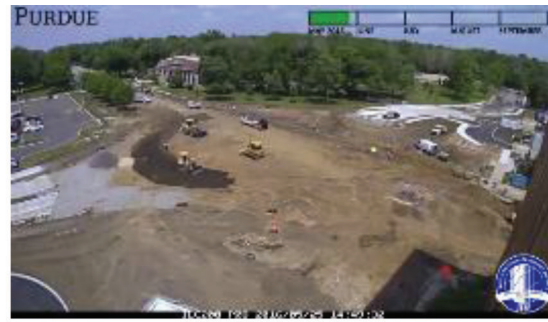
(b) Place subgrade soil for concrete pavement 5/25/16
