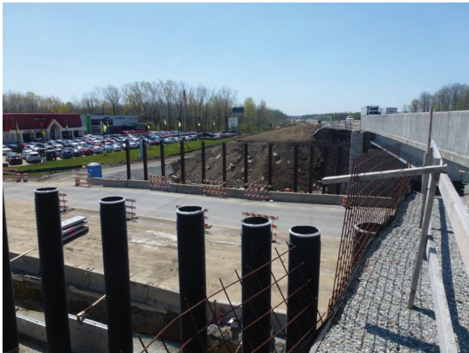
(b) View of uncovered H-piles and covered H-piles from time-lapse camera location
