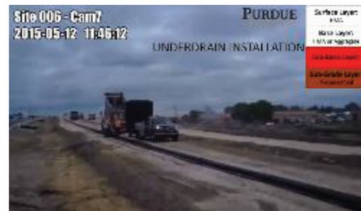
(f) 5/12/15 – Underdrain installation
