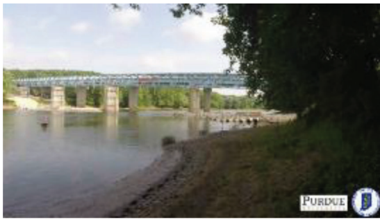
(a) Bridge before charges are set
