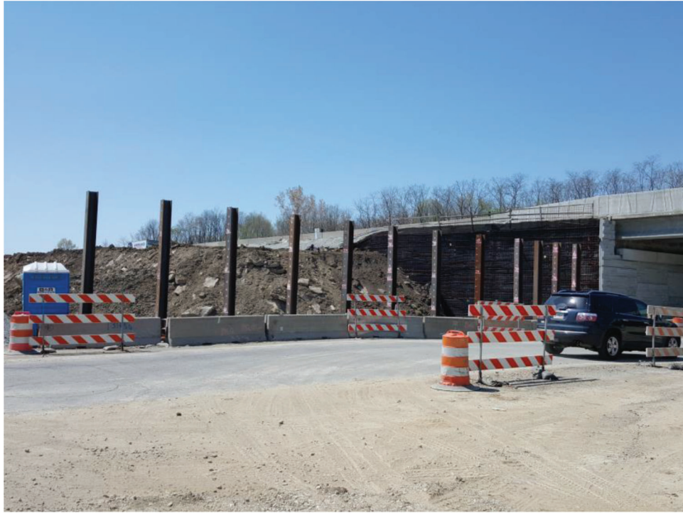
(a) HP 12x74 carbon steel H-piles ground view
