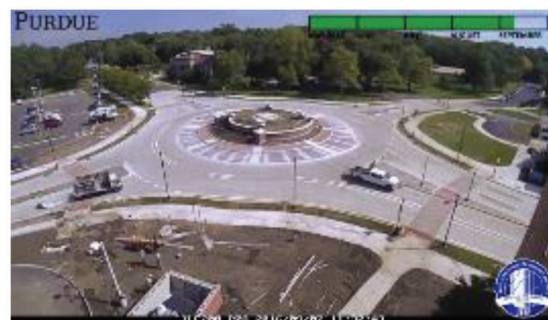
(h) Construct truck apron, lighting, striping, and signage 9/7/16
