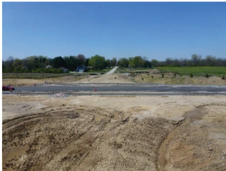
(b) Intersection during construction
