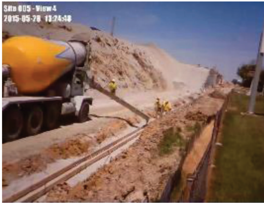
(a) Placing concrete for leveling pad
