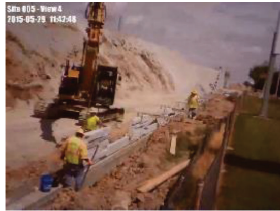
(b) Placing first row of panels
