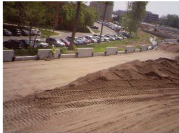
(a) Vibratory plate compactor within 3 feet of wall
