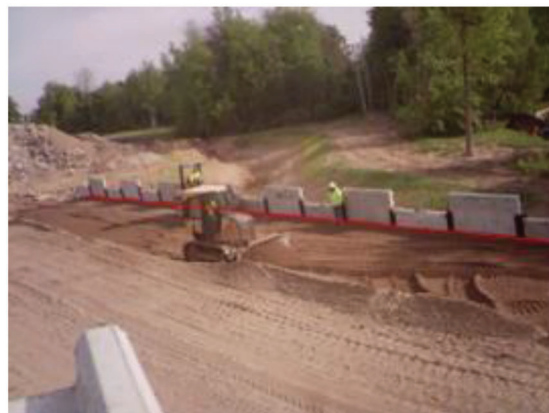
(f) Soil level after lift
