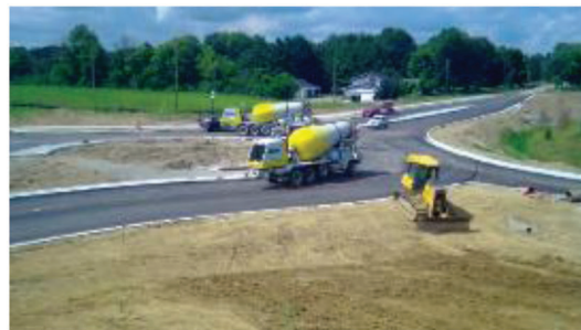
(f) 8/26/15 – Place concrete curbs and truck apron
