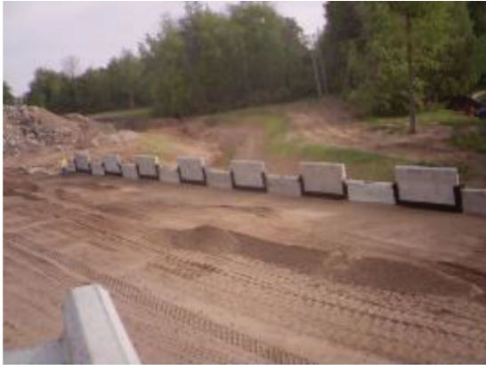
(a) MSE wall ready for next lift of soil
