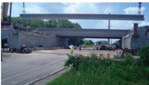
(e) 12:51 PM – Beam is lifted above bridge
