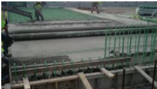
(e) 6/9/15 4:22 PM – Concrete is placed
