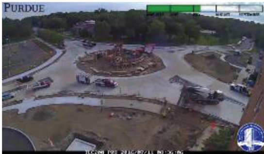
(e) Place concrete sidewalk and construct center piece 7/11/16
