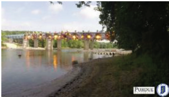
(c) Bridge during implosion
