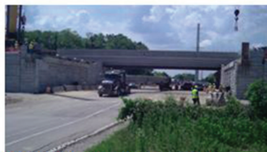
(h) 12:59 PM – Beam No. 9 arrives on site
