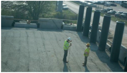
(a) 9:28 AM – Compaction test
