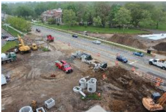
(b) Roundabout during construction
