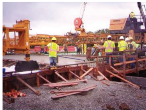
(f) Place concrete deck on bridge 7/9/15
