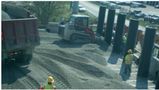
(c) 10:51 AM – Structural backfill placement
