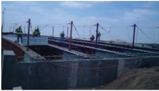
(a) 6/4/15 – Bridge deck pan installation
