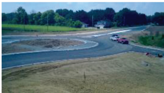
(g) 8/31/15 – Allow concrete to cure
