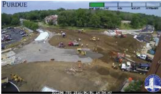
(c) Place aggregate base for concrete pavement 6/1/16
