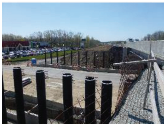
(b) Bridge during construction
