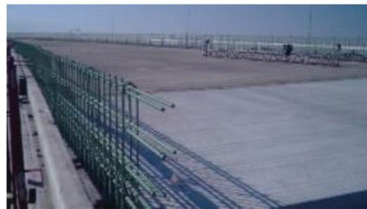
(h) 10/12/15 – Steel layout for concrete guardrail
