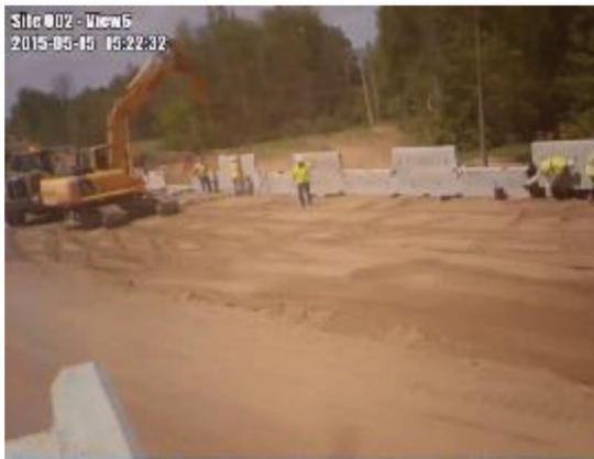
(e) Placing next row of panels
