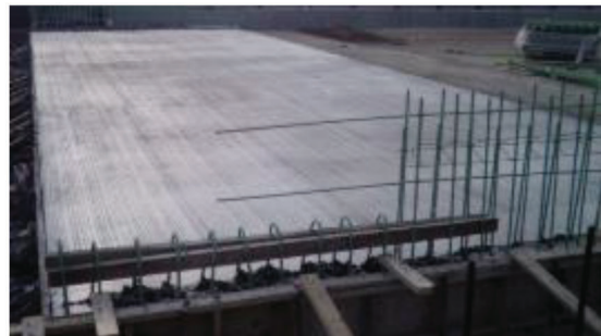
(f) 6/9/15 6:06 PM – Concrete begins to cure
