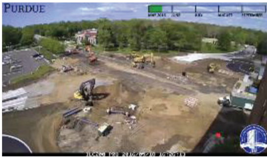
(a) Demolish original intersection 5/18/16
