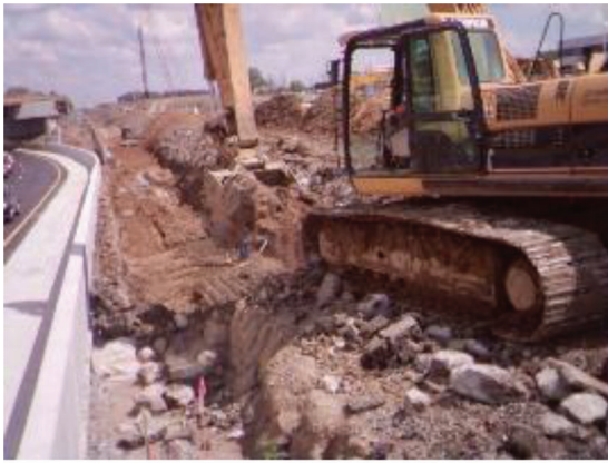
(a) Earthwork for placement of pad
