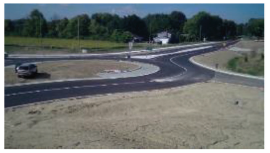
(h) 9/28/16 – Striping, signage, and open to public
