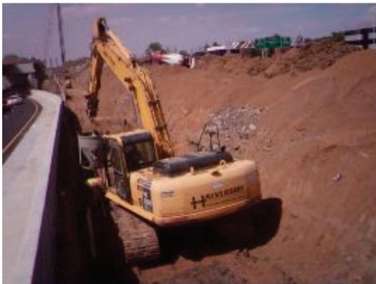
(e) Place leveling pad concrete
