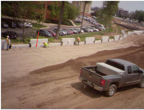
(a) Connecting straps to panels
