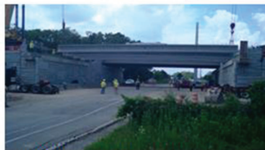
(f) 12:53 PM – Beam is lowered into place
