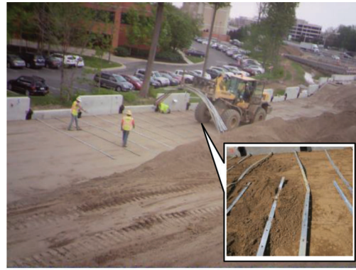
(b) Driving over straps causes damage
