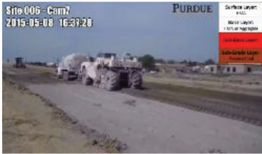
(c) 5/8/15 – Lime mixed into soil
