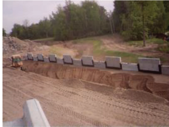
(b) Soil is pushed toward the panels
