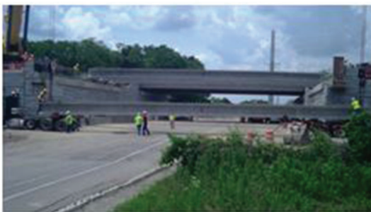
(c) 12:47 PM – Beam No. 8 is attached to cranes
