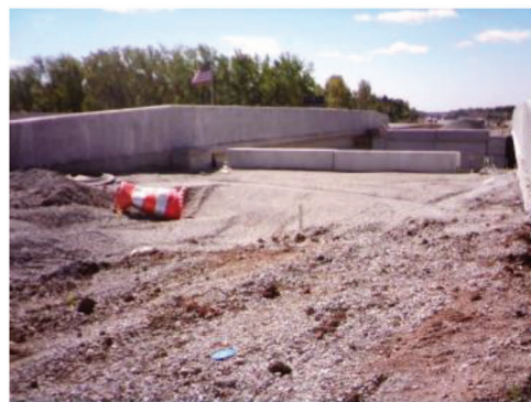
(h) Bridge is complete 8/31/15
