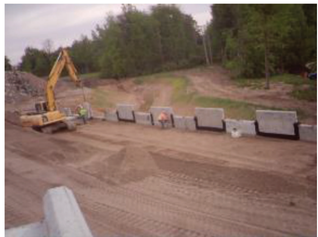
(b) Fabric is placed vertically along the seams
