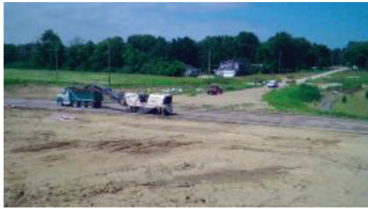
(a) 6/23/15 – Demolition of old roadway
