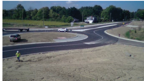
(c) Roundabout construction complete
