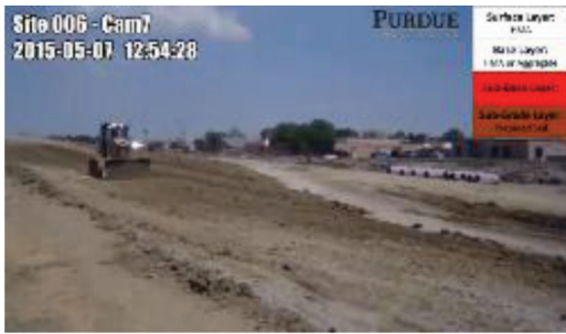
(a) 5/7/15 – Roadway Earthwork
