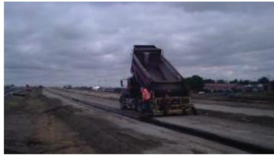
(d) Aggregate placed to facilitate drainage
