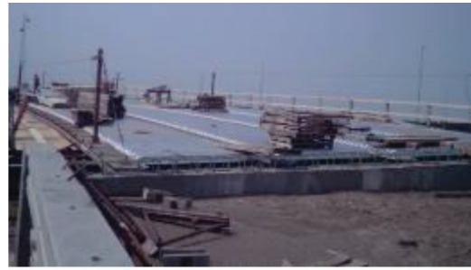
(b) 6/9/15 – Safety railing installed
