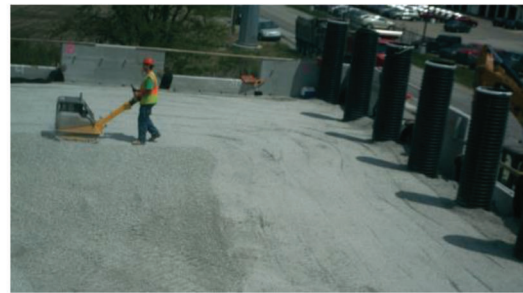
(f) 2:42 PM – Soil compaction
