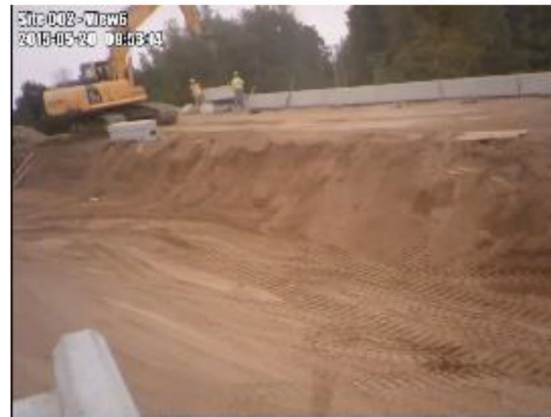
(f) Placing finishing coping
