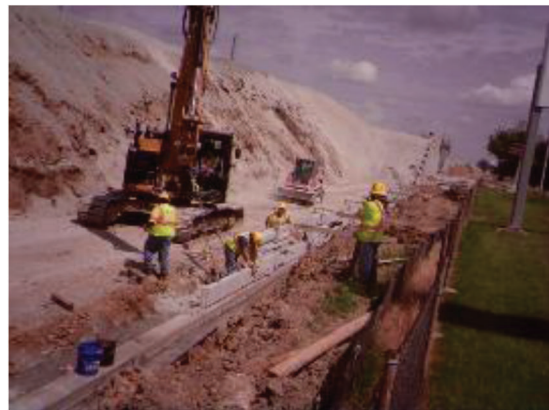
(f) Level half-size panels with wooden shims
