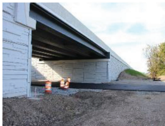
(c) Bridge construction complete
