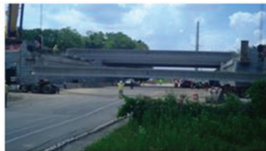
(d) 12:50 PM – Beam is lifted off truck
