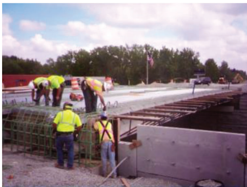
(e) Bridge decking operations 6/16/15
