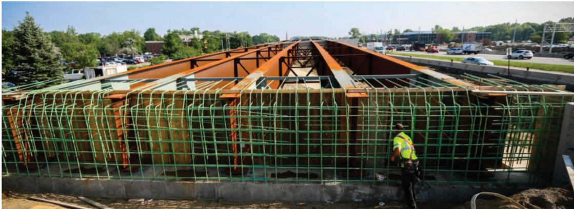
(b) Bridge under construction
