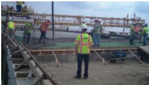
(e) 7/2/15 – Concrete is placed on bridge deck
