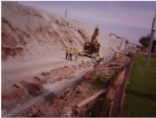
(a) Bare leveling pad – start panel placing
