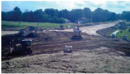
(c) 7/14/15 – Roundabout earthwork
