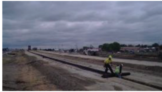
(b) Placing geotextile fabric
