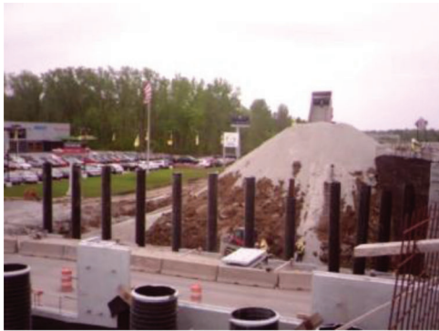
(a) Stockpiling structural backfill 5/14/15
