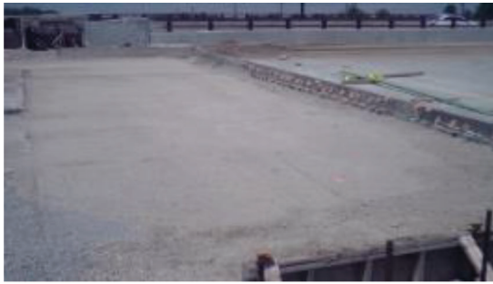
(a) 6/2/15 – Bridge abutment formwork
