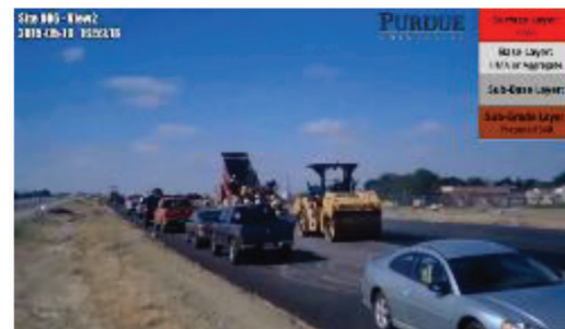
(h) 5/19/15 1:56 PM – Asphalt surface layer is applied
