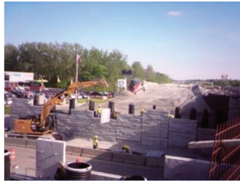
(b) Placing panels of MSE wall 5/19/15
