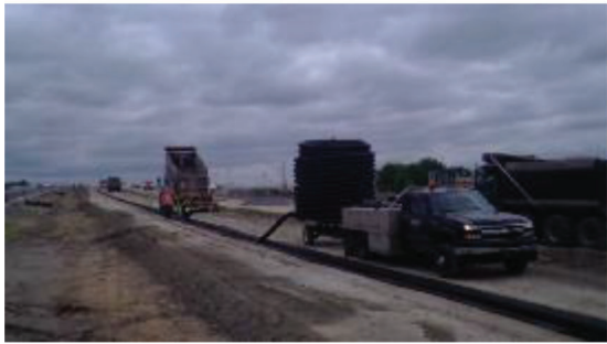
(c) Underdrain pipe placement
