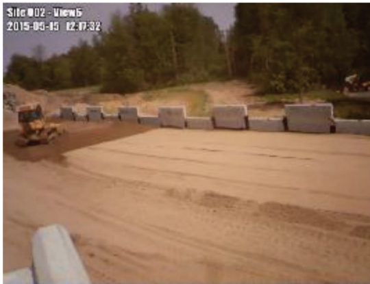
(c) Soil placement – beginning of a lift
