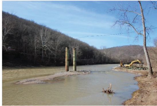
(c) Bridge during removal
