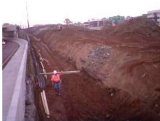
(f) Remove forms and place panels
