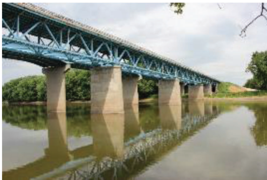
(b) Bridge before demolition
