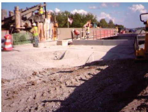
(g) Slip-form concrete guardrails 8/11/15
