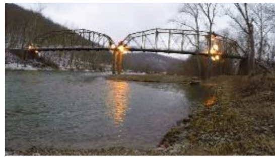
(b) Bridge during implosion
