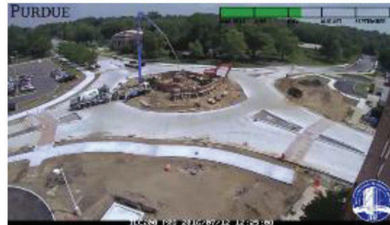
(f) Place concrete at roundabout center 7/12/16
