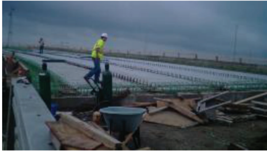
(c) 6/18/15 – Beginning of steel layout
