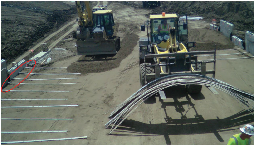
(e) MSE wall ready for next lift of soil
