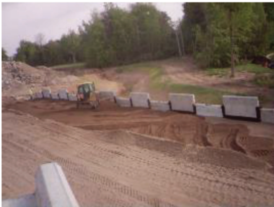
(c) Soil near panels is pushed along the length of the panels
