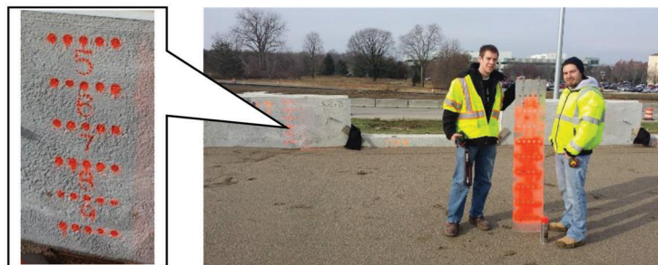
(g) MSE wall backfill lift thickness reference
