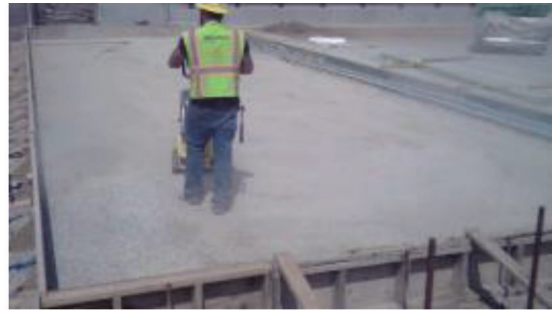
(b) 6/4/15 11:22 AM – Compaction of soil
