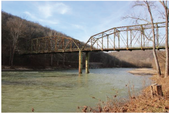
(b) Bridge before retirement
