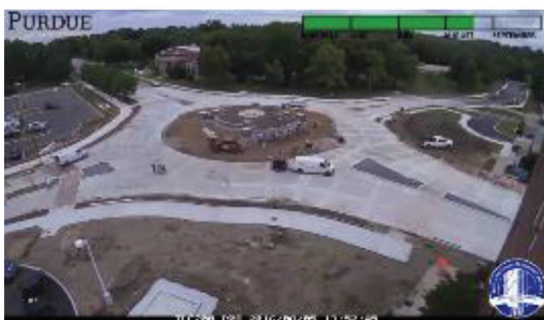
(g) Saw-cut pavement panel joints 8/5/16
