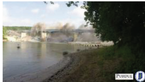
(f) Bridge after implosion
