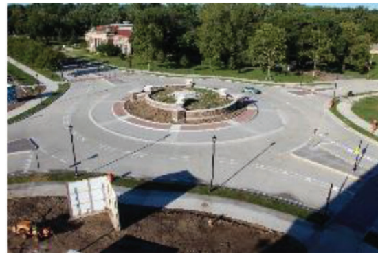
(c) Roundabout construction complete
