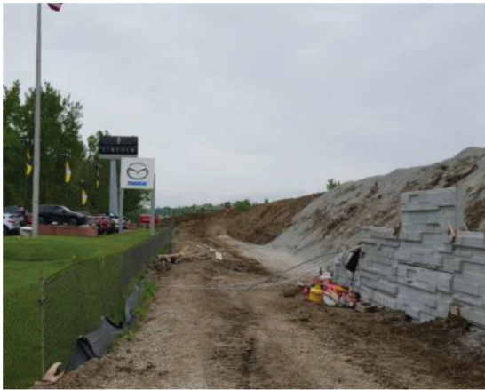
(b) Bridge during construction
