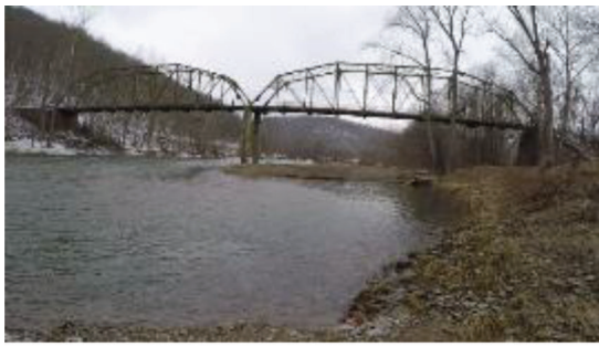
(a) Bridge before charges are set
