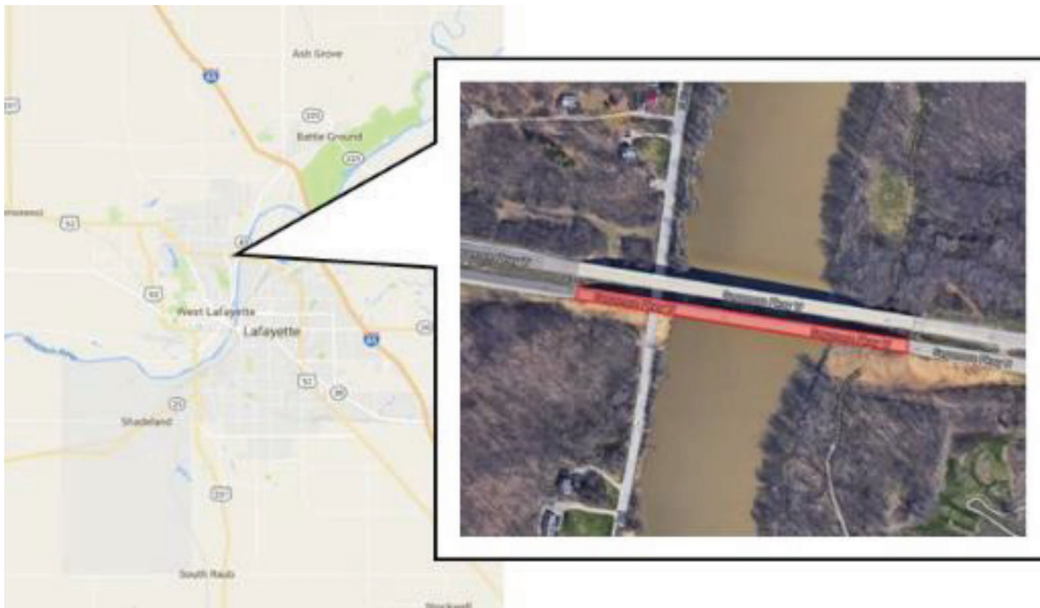
(a) Sagamore Parkway bridge over the Wabash River in Lafayette, Indiana
