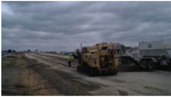
(a) Trench cut for underdrains
