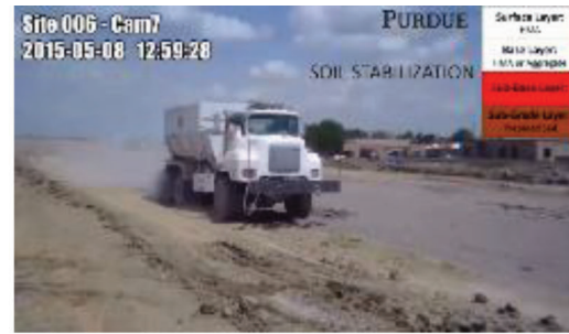
(b) 5/8/15 – Lime soil stabilization
