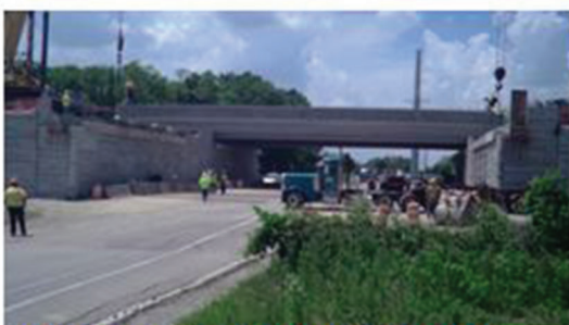
(g) 12:56 PM – Beam is detached from crane
