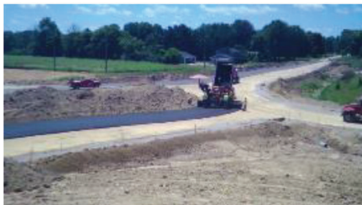
(e) 7/30/15 – Place asphalt base layer
