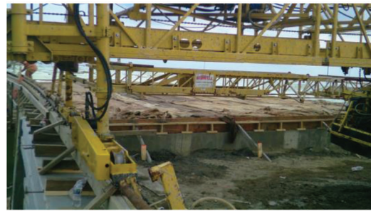
(f) 7/2/15 – Concrete curing under burlap
