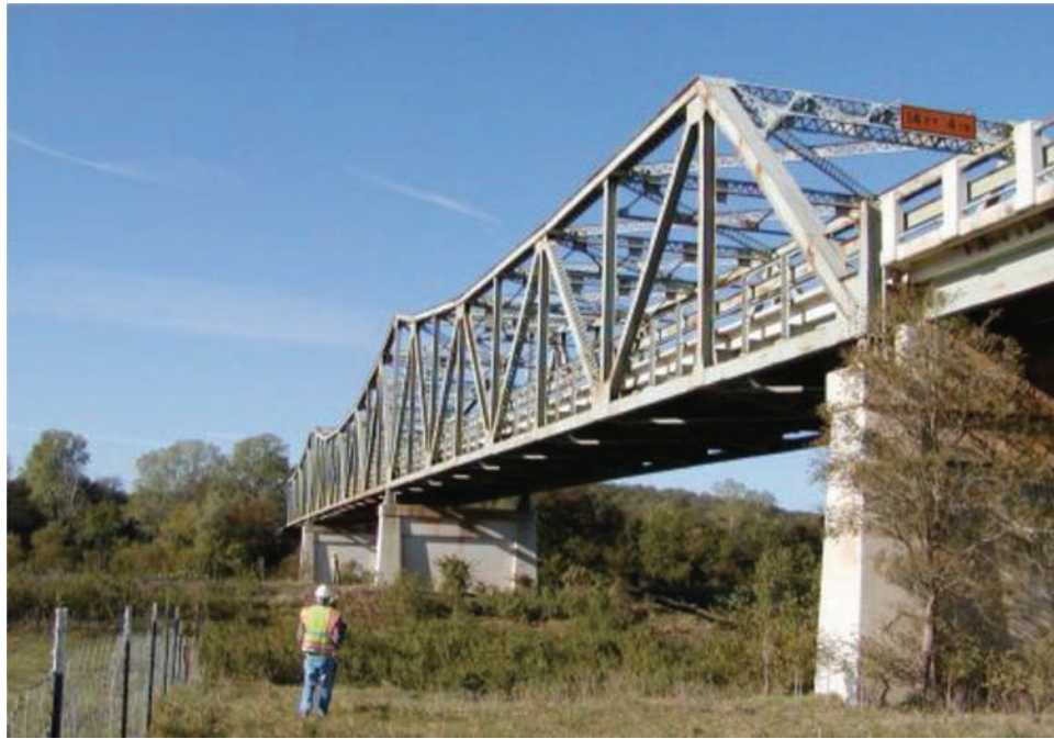
Figure 2.3 U.S. 281 bridge (Buth, 2004).
