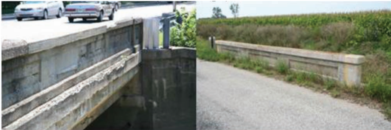
Concrete 1 (Bush-Hammered Panel) (74 bridges)
