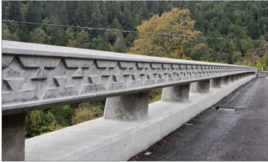
Figure 2.14 Concrete railing with tribal design architectural texture (Caltrans, n.d.).
