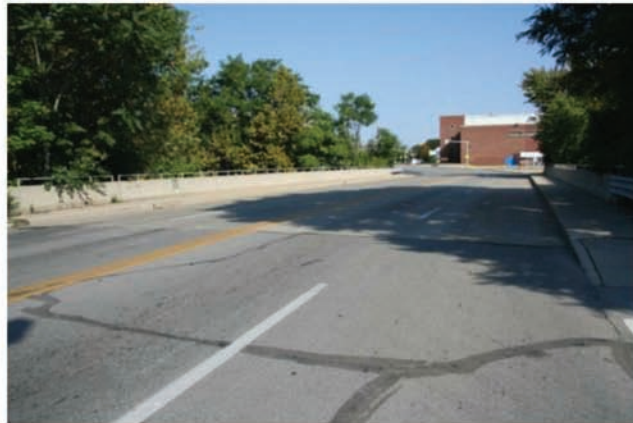
Metal and Concrete 4 (F-type w/ Handrail) (1 bridge)
