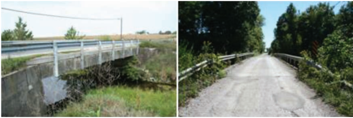
Figure 3.2 Metal 5 (galvanized beam) railing (Rank 2).
