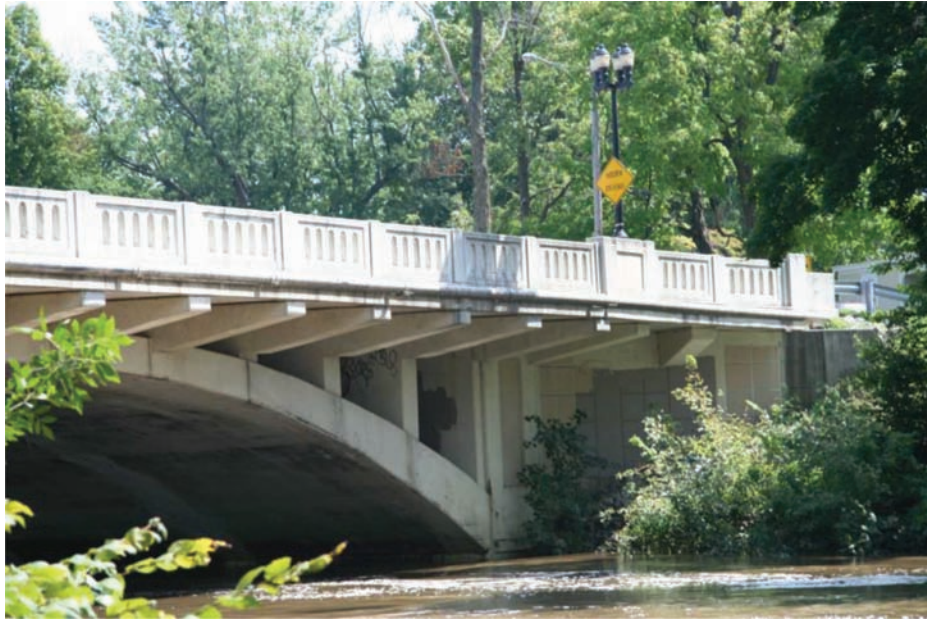
Figure 2.12 INDOT TX railing installation.
