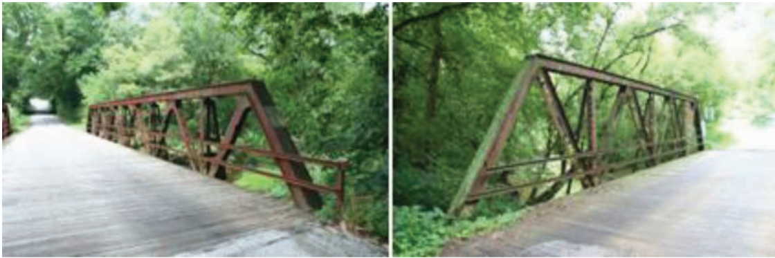
Figure 3.7 Metal 10 railing (Rank 7).
