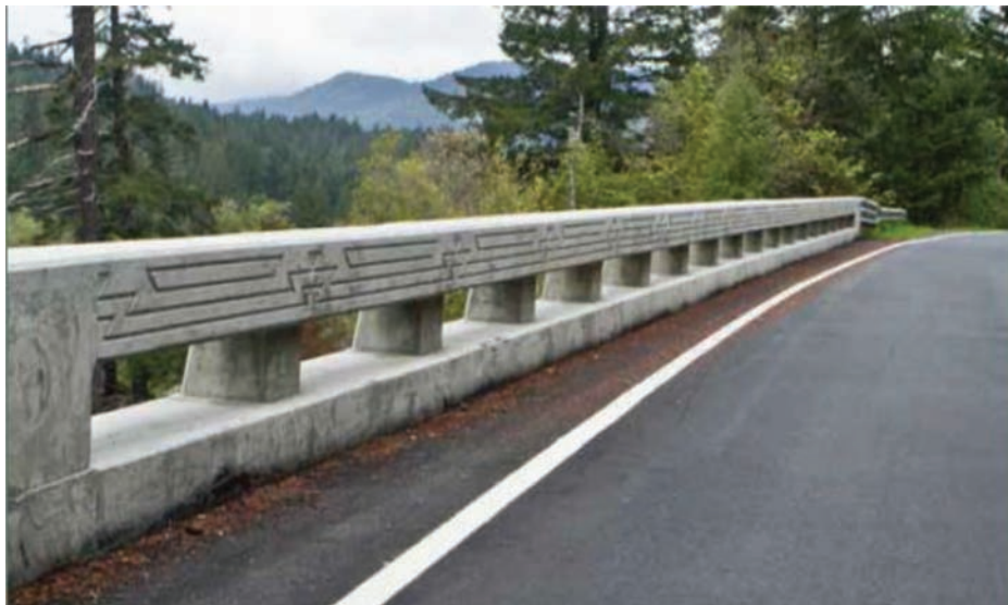
Figure 2.13 Concrete railing with tribal design architectural texture (Caltrans, n.d.).
