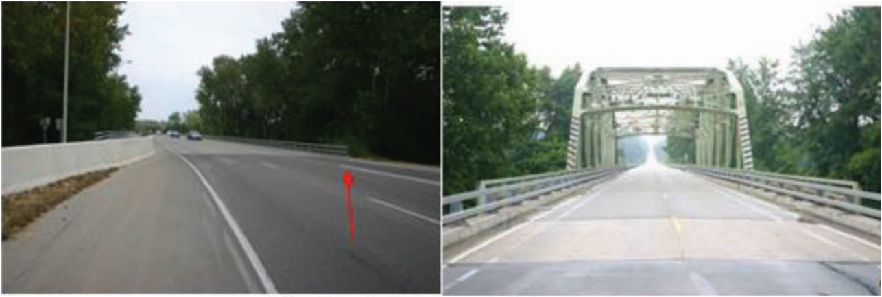
Metal and Concrete 2 (2 bridges)
