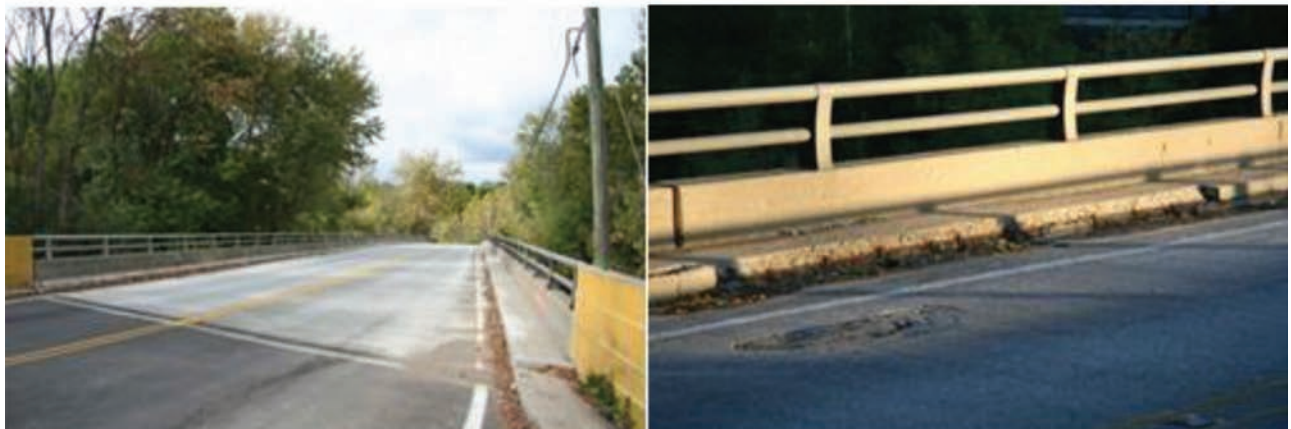
Metal and Concrete 1 (8 bridges)
