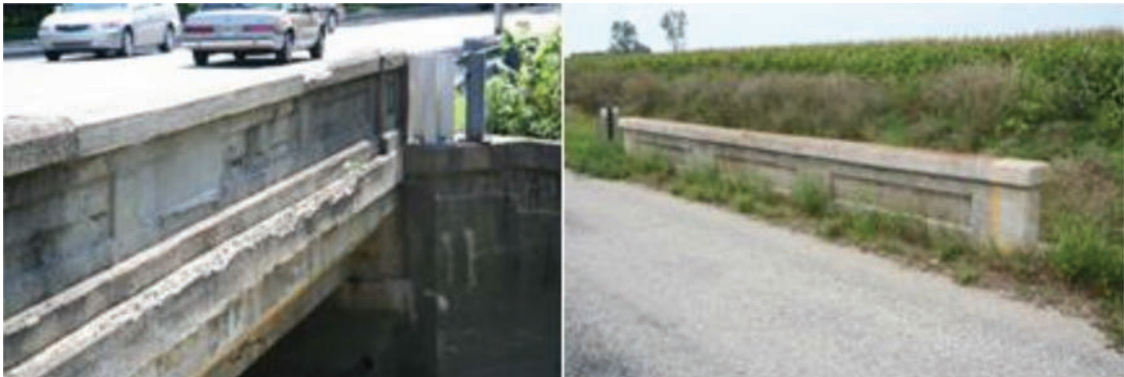
Figure 3.3 Concrete 1 (bush-hammered panel) railing (Rank 3).
