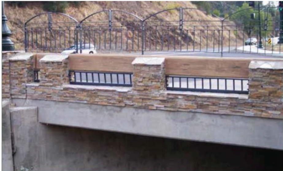
Figure 2.15 Concrete railing with architectural treatment (Caltrans, n.d.).
