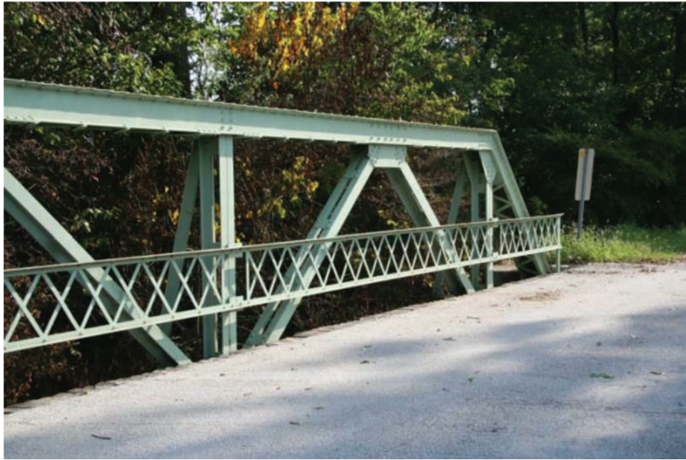
Figure 4.24 Metal 6 railing on historic pony truss bridge.
