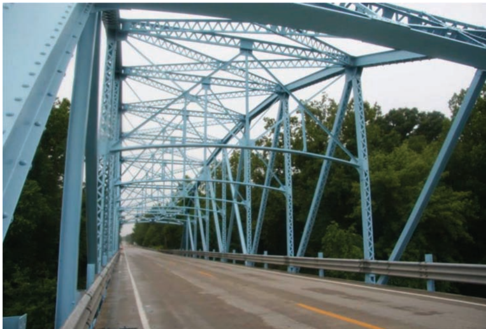
Figure 4.21 Metal thru truss with a railing ineligible for replication.
