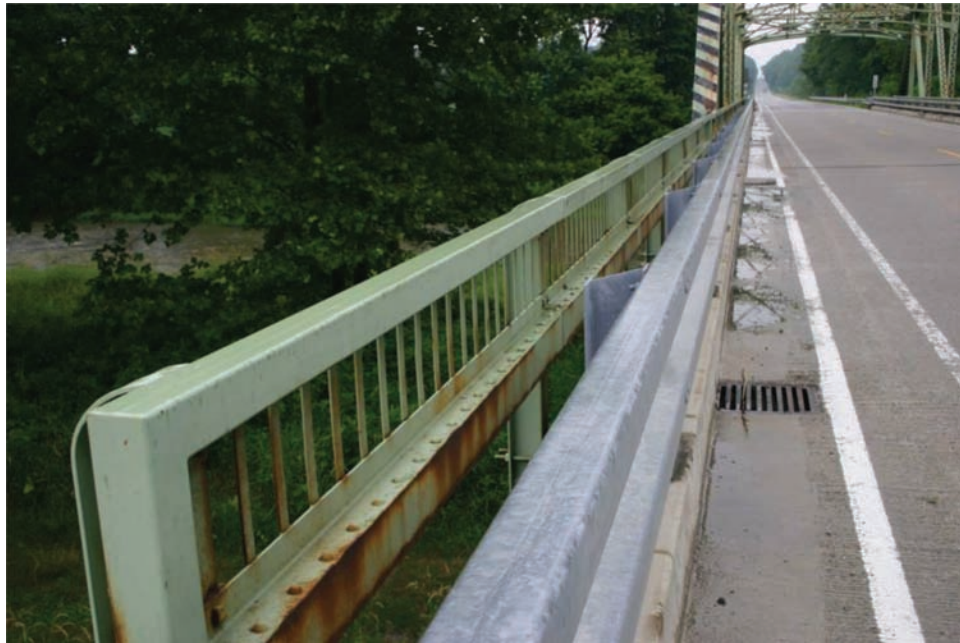
Figure 4.22 Close-up of Metal 14 railing (light green).
