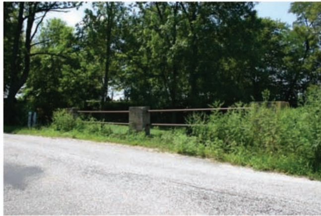
Metal and Concrete 3 (1 bridge)
