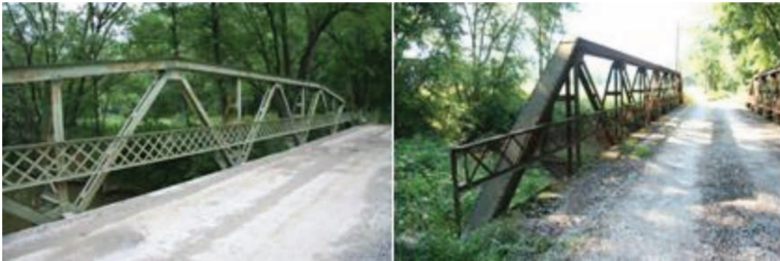
Figure 3.1 Metal 6 railing (Rank 1).
