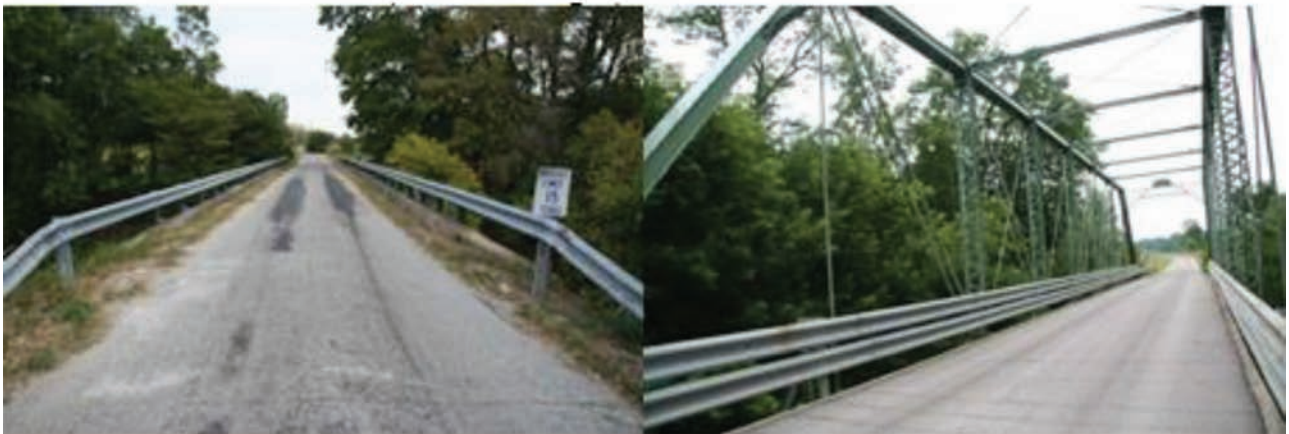
Metal 5 (Galvanized Beam) (75 bridges)
