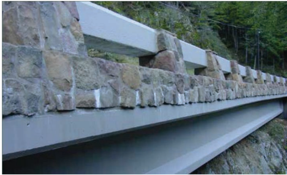
Figure 2.16 Concrete railing with architectural treatment (Caltrans, n.d.).
