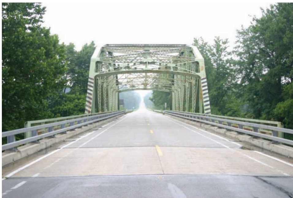
Figure 4.2 A metal thru truss with an inboard railing.
