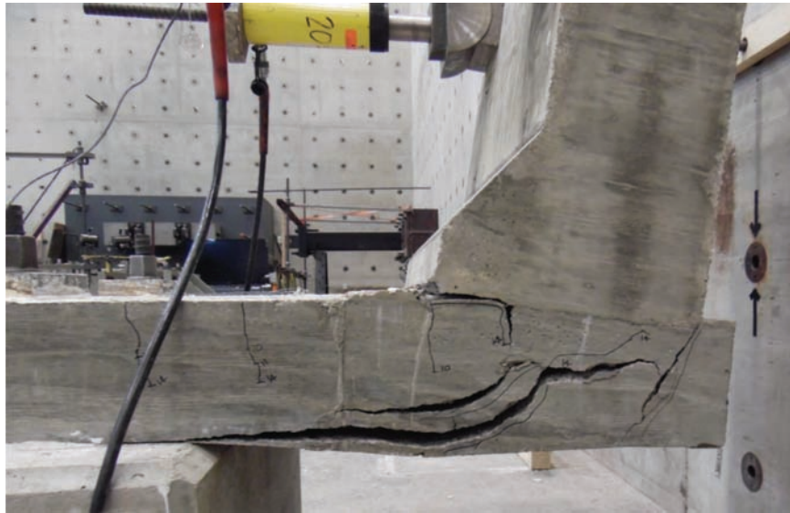
Figure 5.21 Strip Specimen 1 failure plane at 14 kip.
