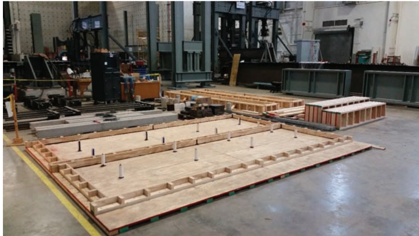
Figure 4.7 Completed Specimens 1 and 2 formwork.
