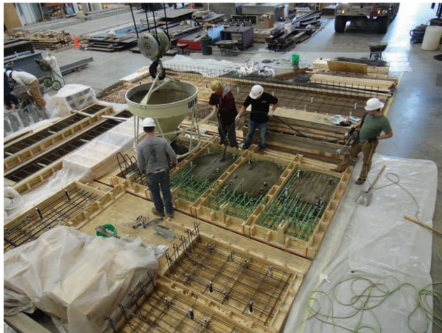
Figure 5.4 Strip specimen slab cast.
