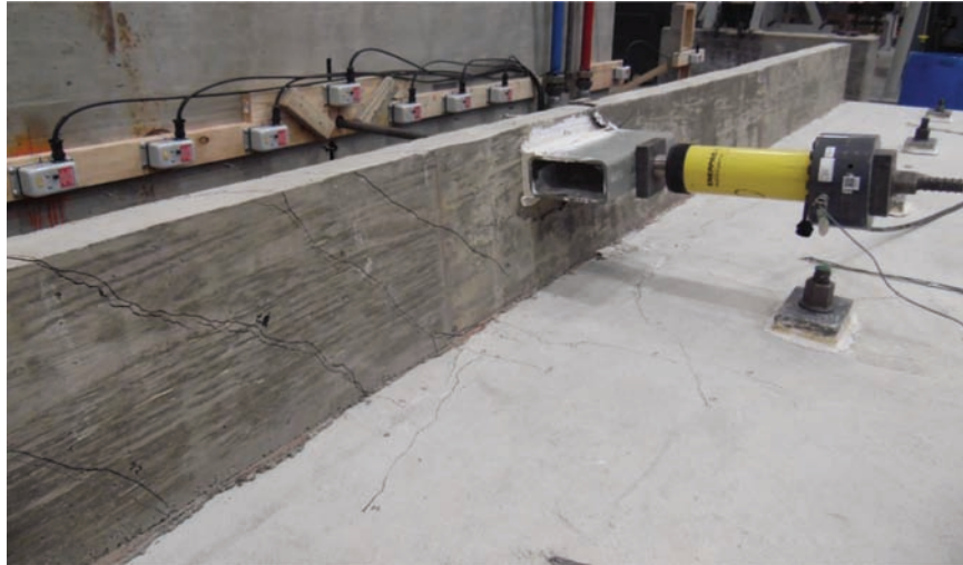
Figure 4.45 Punching shear failure (Specimen 1L).
