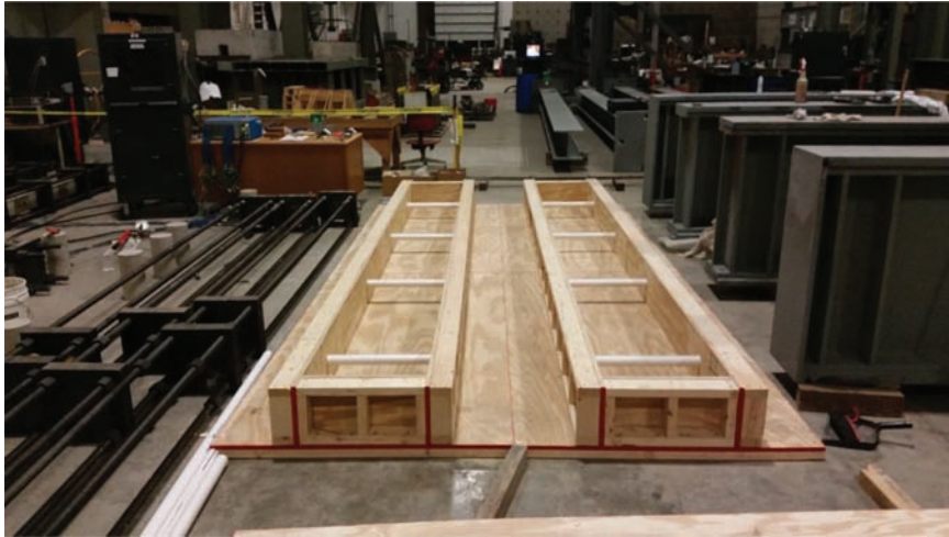
Figure 4.8 Completed support beam formwork.
