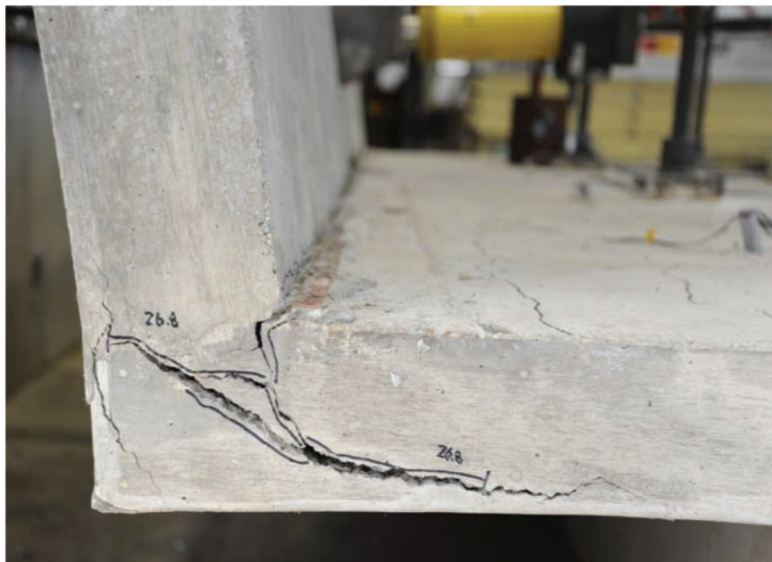
Figure 4.35 Diagonal tension failure (Specimen 1).
