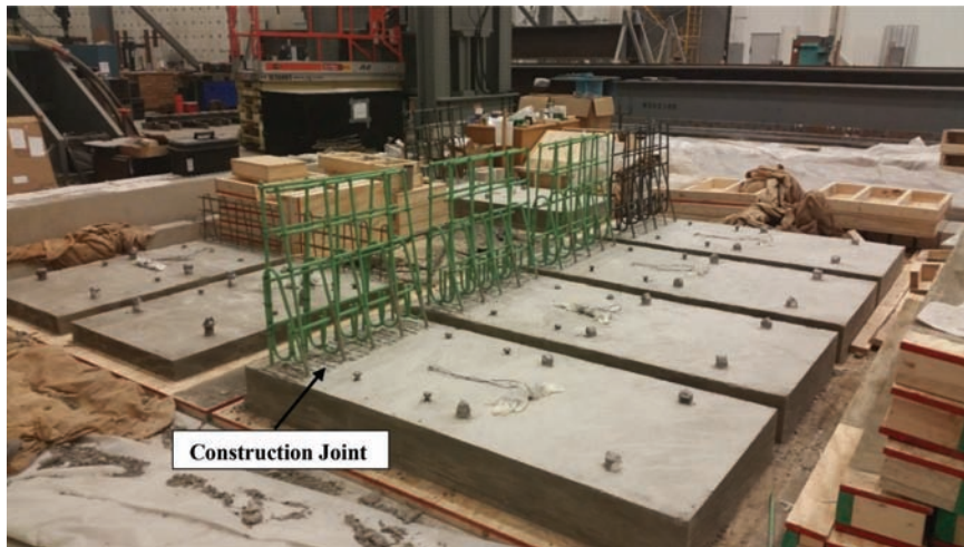
Figure 5.6 Barrier reinforcement for strip specimens.
