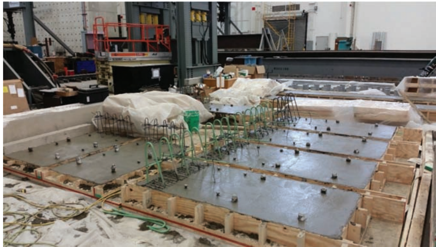
Figure 5.5 Completed strip specimen slab cast.
