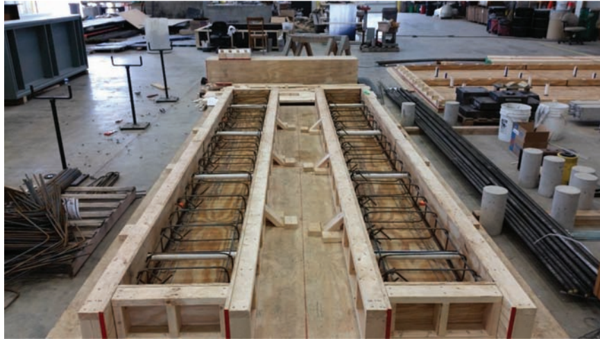
Figure 4.11 Reinforcement in support beams.
