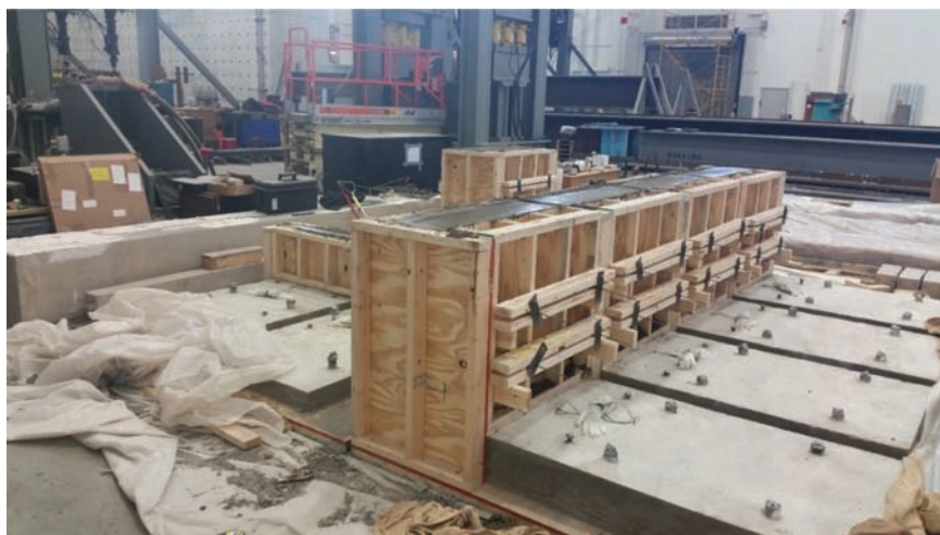
Figure 5.7 Completed barrier cast.
