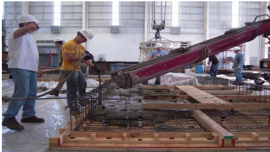
Figure 4.12 Slab cast (Specimens 1 and 2).
