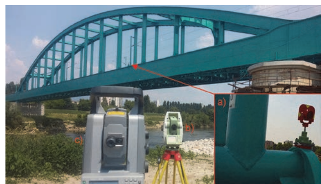
Figure 2. Position of RTS instruments and reflector; a - reflector; b - RTS 1; c - RTS 2
