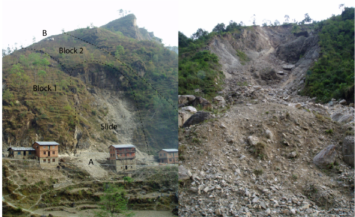
Figure 4.12 Left - The active translational slide in Chaku. Five houses were destroyed by a landslide in 2001 (A). A house remains occupied above the main scarp of the landslide (B) which is retrogressing up the hillslope putting more houses at risk. Right – A colluvial fan at the bottom of Chaku settlement. Evidence of secondary lateral slumping can be seen.
