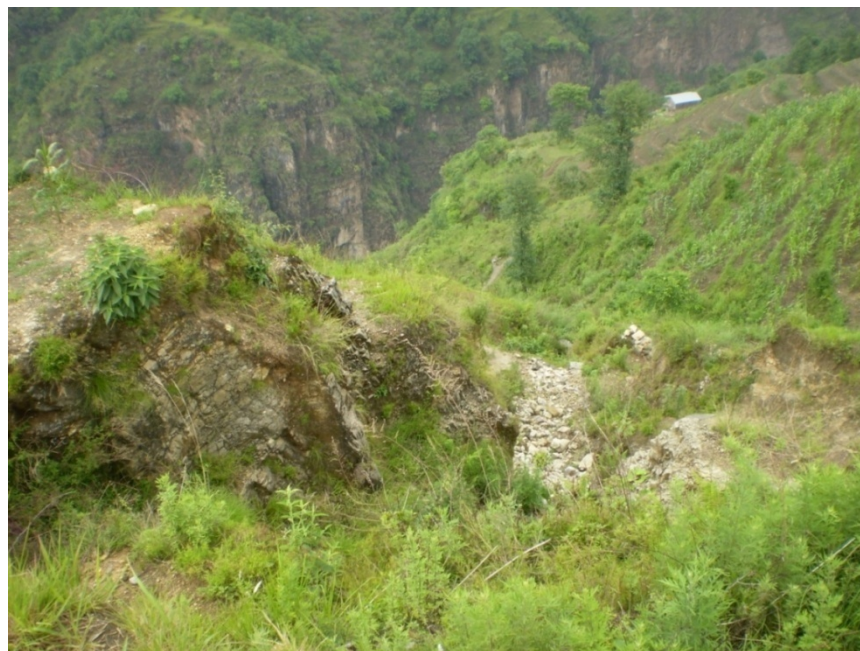
Figure 4.20 Terraces destroyed by the active translational slide at the bottom of Marmin settlement.
