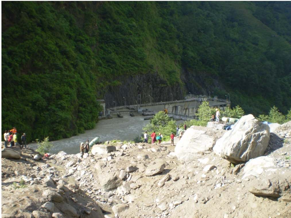
Figure 4.17 The Tatopani debris flow reactivated following heavy monsoon rains in July 2007. Landslide material partially blocks the Bhote Koshi River behind the Tatopani hydropower dam.
