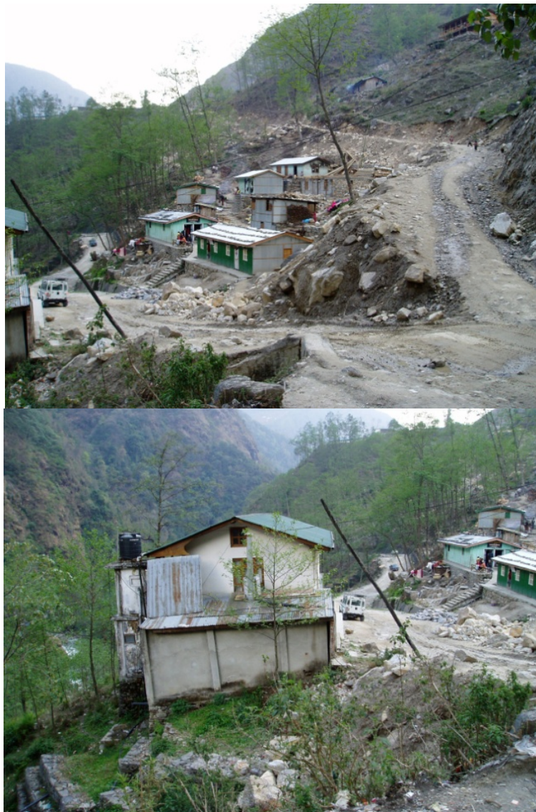
Figure 4.19 The roadside settlement of Kodari. Inclining trees, marked changes in the level of the road and cracks in the Eco Hotel (bottom photograph) are indicators of continuous slope movement.
