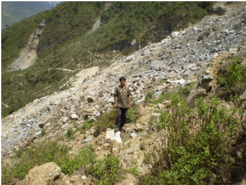
Figure 4.23 The 2006 Chambang landslide.
