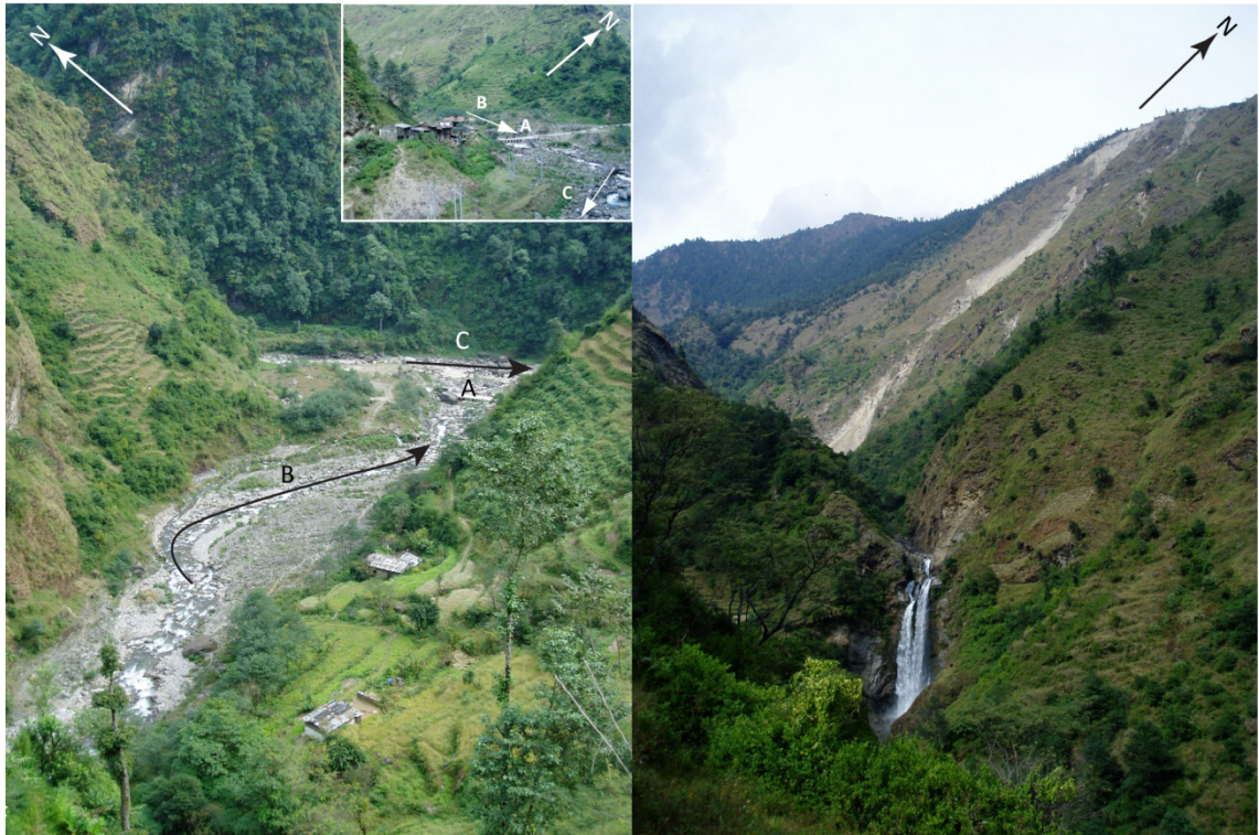
Figure 4.15 Left - The Bhairab Kunda Khola. Extensive aggradation and erosion caused by the 1996 channelised debris flow resulted in the loss of farmland and the lateral migration of the stream channel. The Bhairab Kunda Khola (B) joining the Bhote Koshi River (C) below Larcha bridge (A). The inset shows the settlement of Larcha at the confluence of the Bhairab Kunda Stream and the Bhote Koshi River. Right – An active gully depositing material into the Bhairab Kunda Khola approximately 750 m upstream from Larcha.
