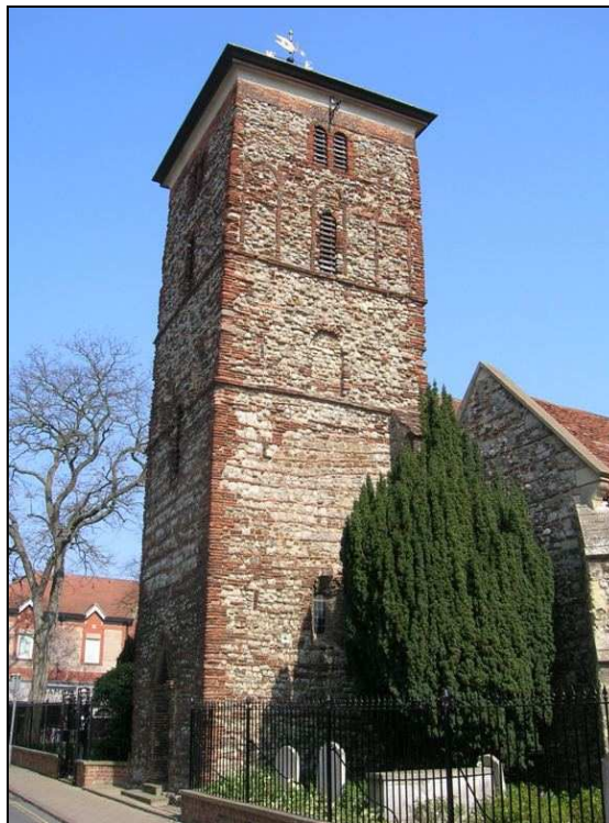
Fig. 2.10: Western tower of Holy Trinity church, Colchester. Note the red quoins, string courses, horizontal banding and blind arcading of the upper stages, all made from brick robbed from surrounding Roman buildings.
