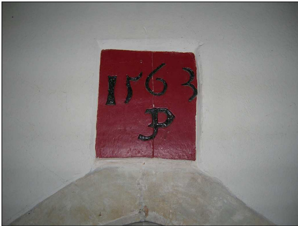
Fig. 3.120: Date plate of 1563 within Woodham Walter church.
