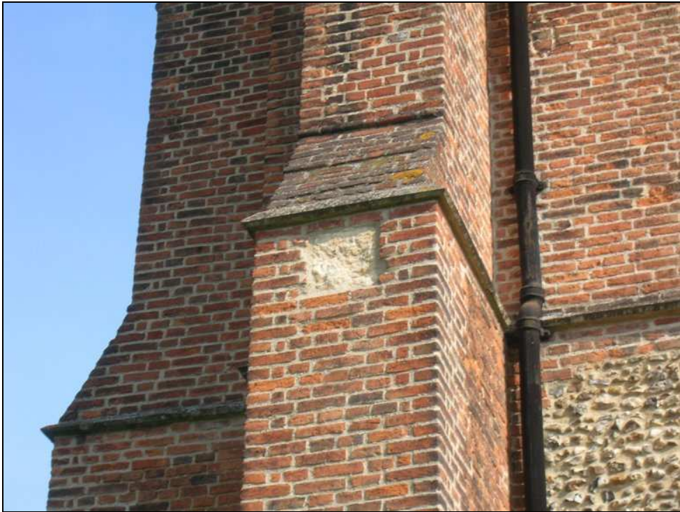
Fig. 3.100: Stone inset into the brick buttress on the southern face of the tower at the top of the first stage. Antiquarian accounts record that the Mildmay family arms and the date 1586 were originally inscribed in the stone.
