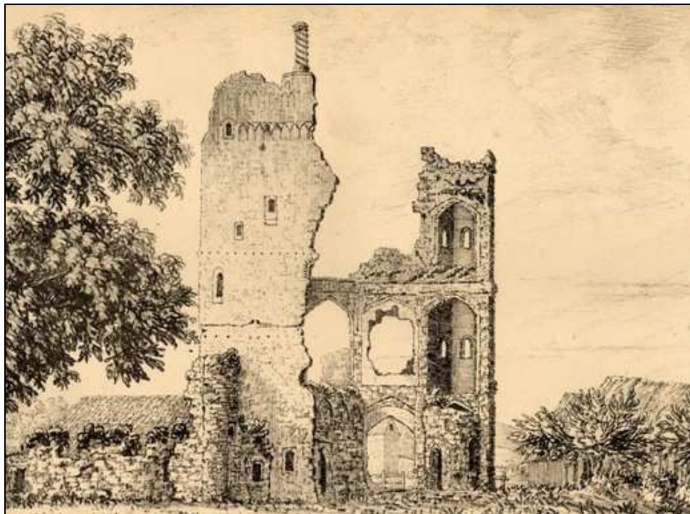
Fig. 3.42: Sketch of Nether Hall gatehouse made in 1819 from the north inside the moated complex (ERO I/Mb 302/1/6).
