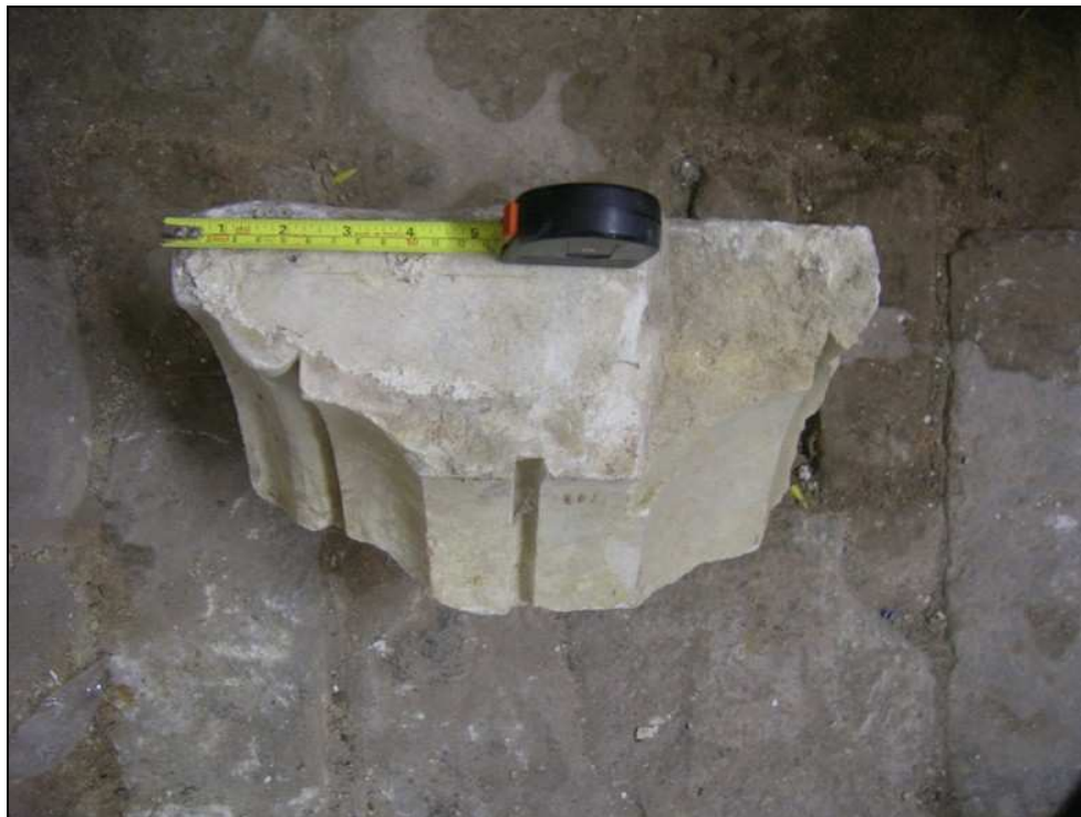
Fig. 3.59: Part of a window spandrel that had been re-used as a flag in the cellar floor. The top image shows the ogee and quarter circle moulding beneath the spandrel whilst the bottom image shows the cross sectional profile.
