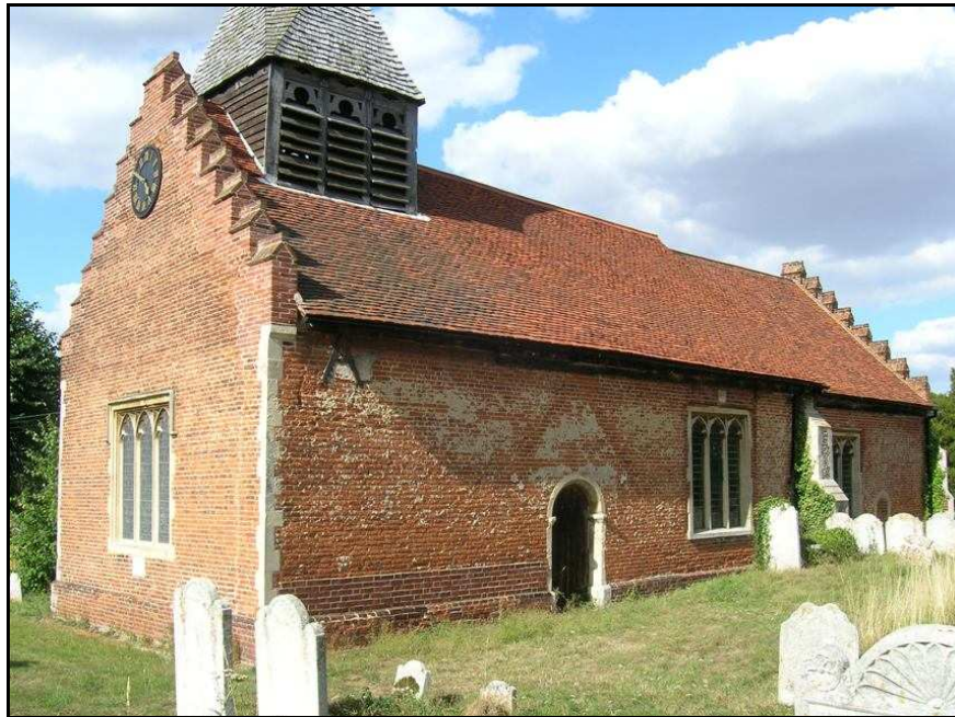
Fig. 3.119: St. Michael’s church, Woodham Walter, from the south west corner. Note the traces of plaster on the southern wall and the outline of the earlier porch roof above the southern door.
