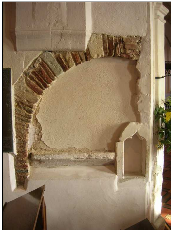
Fig. 3.72: Small niche in the wall north of the opening between the nave and tower. The pattern of construction (brick and stone voussoirs) is the same as the original chancel arch (see Fig. 3.71).
