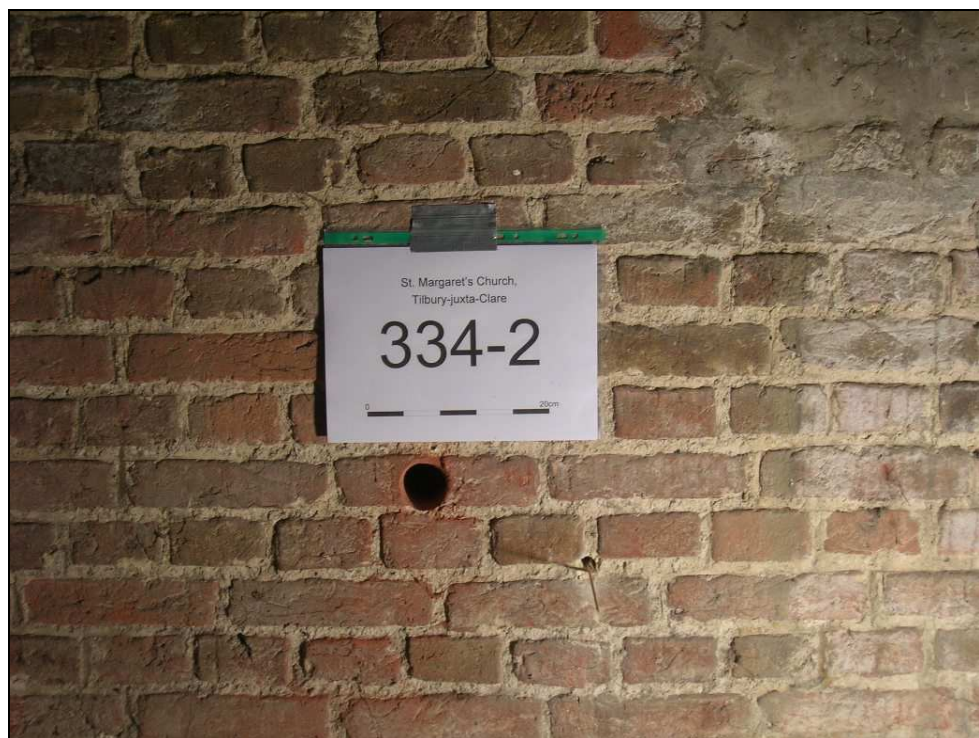
Fig. 3.118: The sample point in the northern wall of the church tower. The scale is 20 cm in length.
