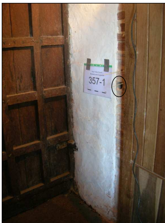
Fig. 3.78: The sampling point on the brick quoin of the southern doorway inner order, seen on the right of the image (the sampling point is circled). The scale bar is 20 cm in length.
