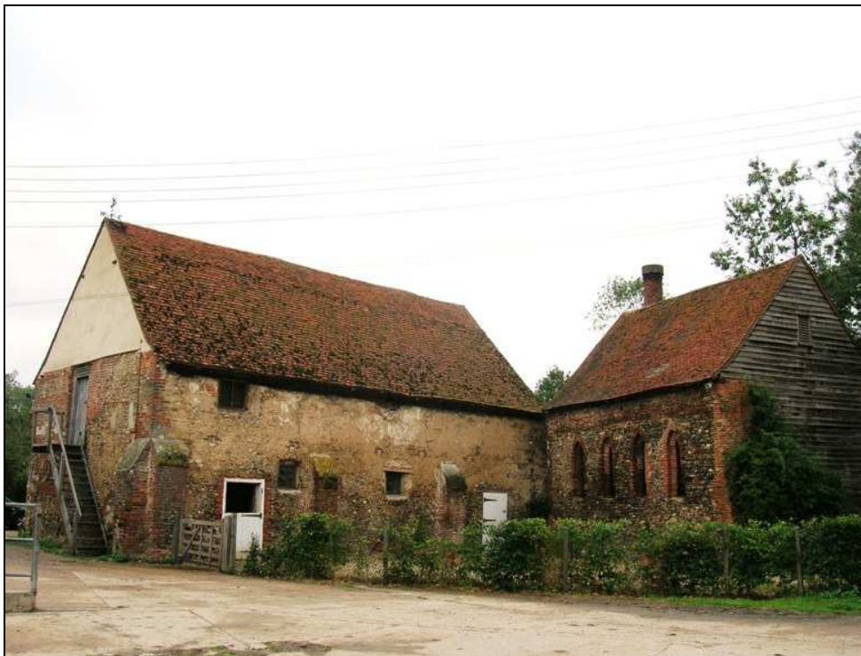
Fig. 3.6: View from south west of two monastic buildings. That on the left is thought to be the abbot's lodgings whilst the building on the right is thought to be the guest house.
