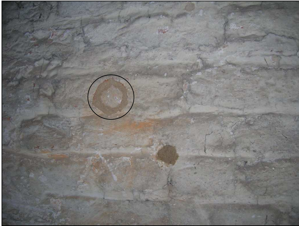
Fig. 3.83: The sampling point (circled) at St. Andrew's church. The sample and dose capsule hole (below and to the right of the sampling point) have both been filled with lime mortar.
