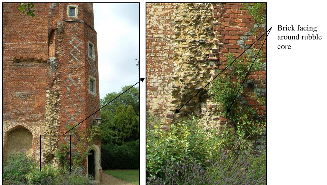
Fig. 2.18: Brick facing around rubble core on south eastern corner of the inner courtyard gatehouse at Leez Priory.
