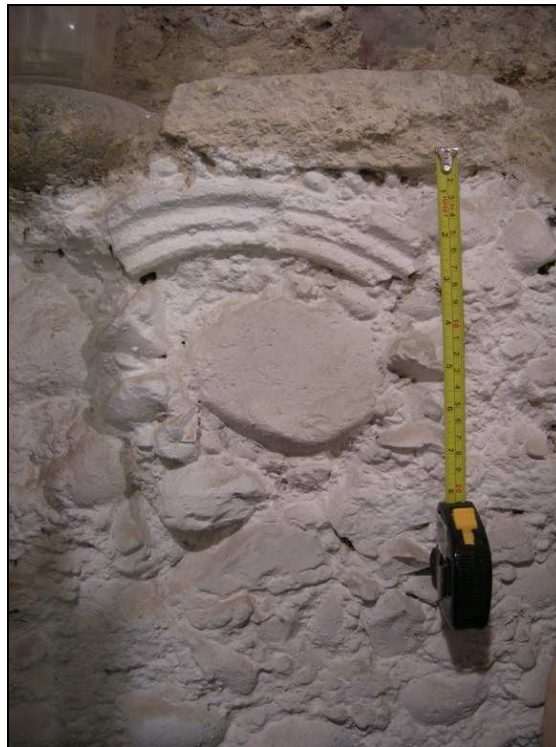
Fig. 3.93: Fragment of carved stone reset in the rubble walling of the sunken chamber (the tape measure is extended 20 cm).
