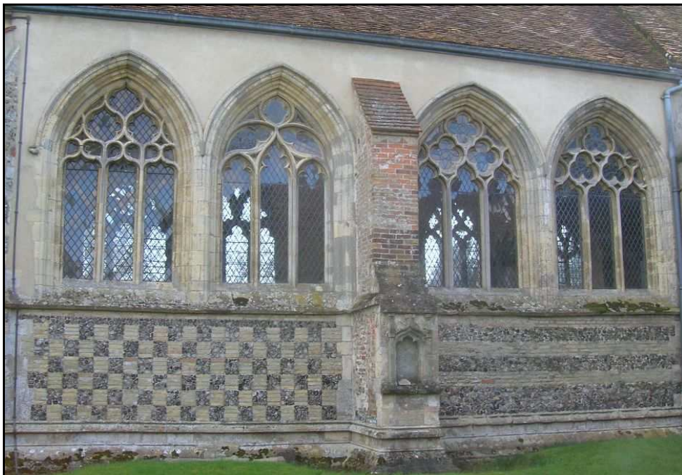
Fig. 2.13: North face of Lawford chancel showing two different decorative uses of yellow Flemish type brick: chequer-work with knapped flint (left) and horizontal bands of alternating brick and knapped flint (right).
