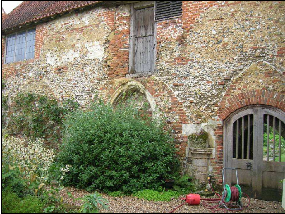
Fig. 3.4: Evidence of sub-dormitory vaulting at southern end of eastern cloister range. Note the wallshaft with moulded capital and keying marks for the quadripartite vaulting to the underside of the dormitory.
