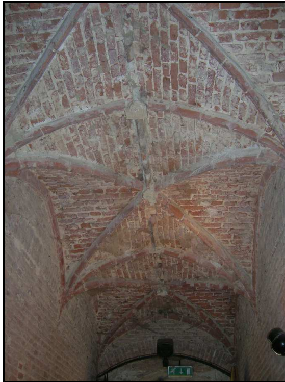
Fig. 3.43: Brick quadripartite vaulted entrance passageway inside Rye House gatehouse. Whilst the vaulting at Nether Hall has fallen in, there is evidence that the passage was originally vaulted in three bays.
