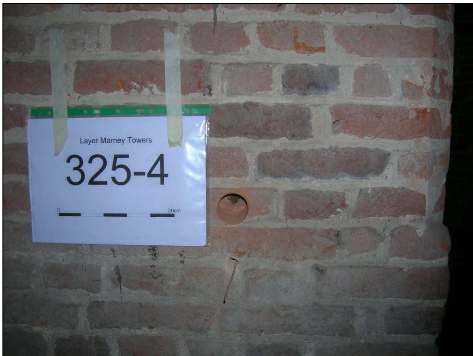
Fig. 3.29: The brickwork at the sampling point in Layer Marney. The scale bar is 20 cm in length. A door jamb can be seen to the right side of the image.
