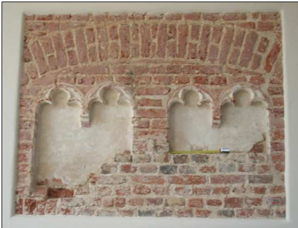
Fig. 3.36: Decorative trefoil corbelled niches made from carved, ruddled bricks above the fireplace within the Moot Hall.
