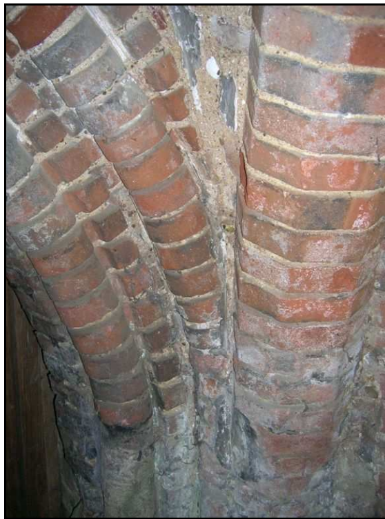
Fig. 2.3: Springing for a roll moulded doorway (left) and a chamfered vaulting rib (right) at Coggeshall Abbey.
