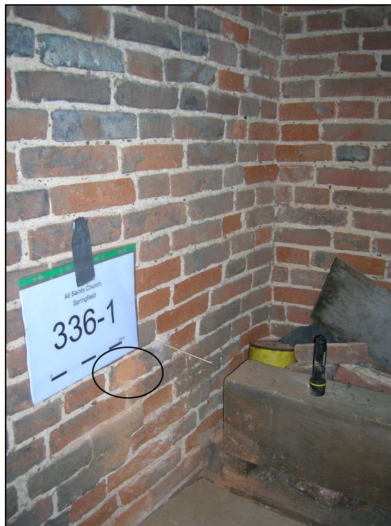
Fig. 3.102: The sampling point in the tower belfry, close to the south west corner. The scale is 20 cm in length and the sampling point is circled. Note the irregular bonding pattern of the brickwork. There is also a high degree of variation in the colour of the 'Tudor' bricks, ranging from orange to a dark blue and black.
