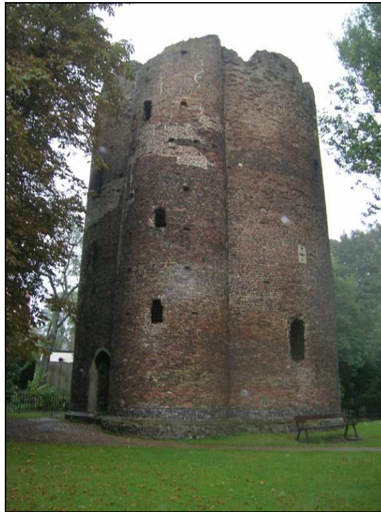
Fig. 2.6: The Cow Tower in Norwich, showing an early example of brick being used specifically as a dressing material.
