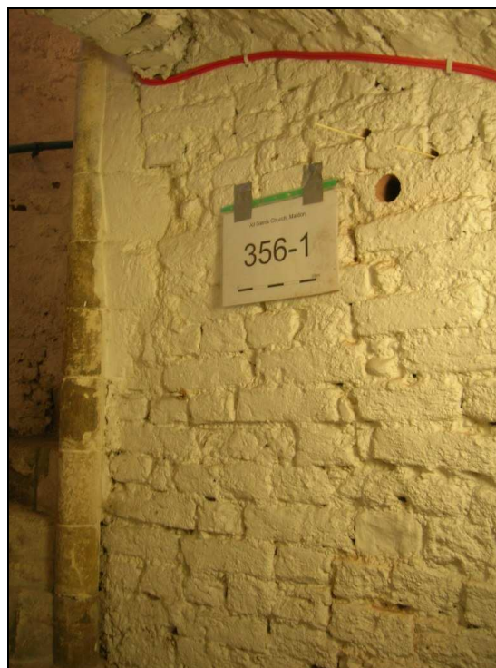
Fig. 3.97: The sampling point in the western wall on the lower stage of the staircase leading down into the sunken chamber. The scale is 20 cm in length.
