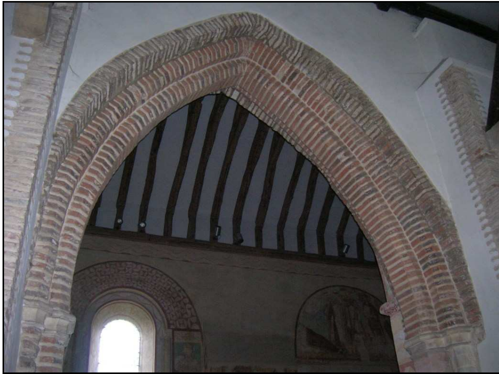
Fig. 2.11: Late 13 th century lancet at Copford church. The outer order brickwork is re-used Roman whilst the two inner two orders are medieval.
