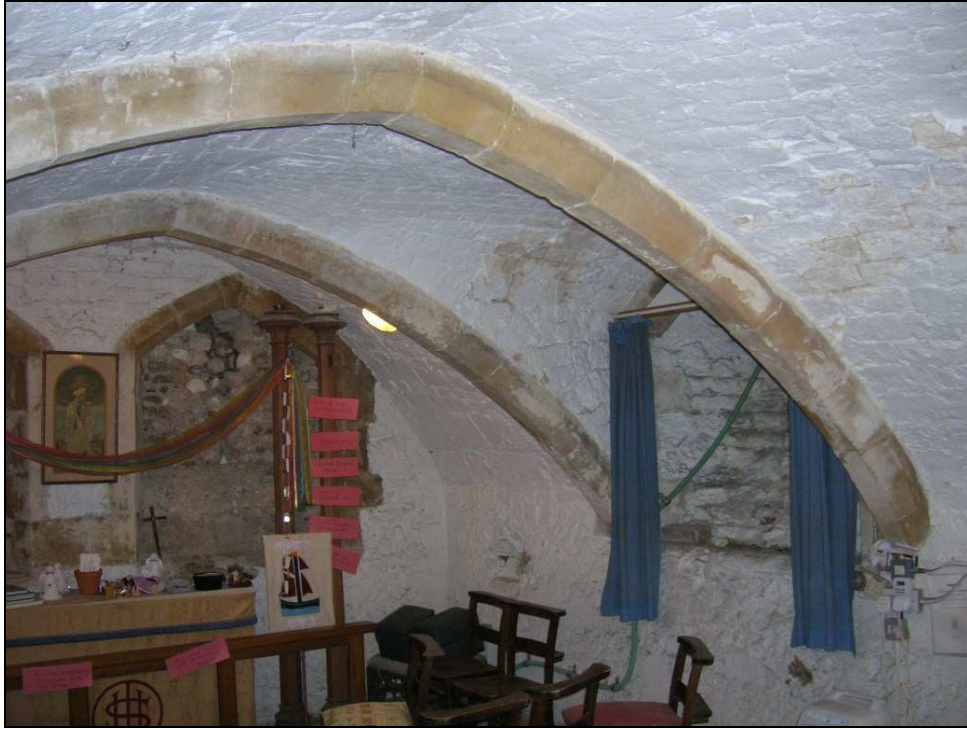
Fig. 3.92: The sunken chamber of All Saints' church. Note the two blocked openings at the east end of the chamber (left side of the image), the transverse ribbed arches and the splayed window in the southern wall (right side of image).
