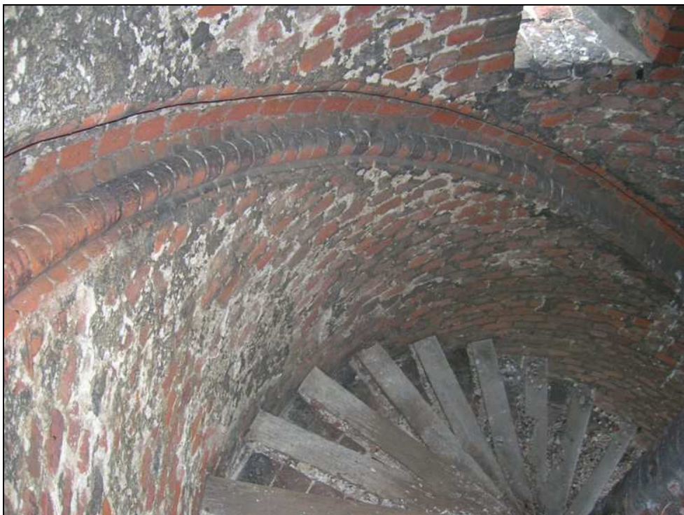
Fig. 3.44: The view down the brick newel staircase, illustrating the header bonded wall and the moulded brick handrail laid in header fashion.
