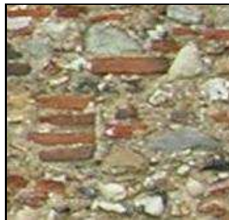
Fig. 6.1: Fairstead church chancel. The current chancel end is thought to have been extended in the 13 th century, possibly replacing an earlier structure. The quoins that identify the eastern extent of the earlier structure are preserved in the wall fabric and are circled in the main image. Coggleshall type brick occurs randomly among the flint rubble walling of the 13 th century square eastern end, an example of which is shown in the bottom image where Coggleshall type bricks have been used to form part of a put log hole. The occurrence of Coggleshall type bricks in the later 13 th century chancel suggests re-use from an earlier context.
