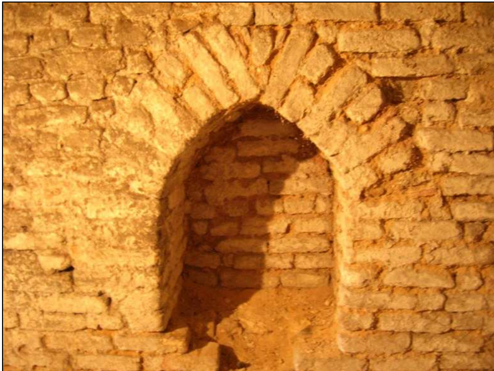
Fig. 3.64: The alcove in the west end of the cellar. The arch would suggest an early 14 th century date.
