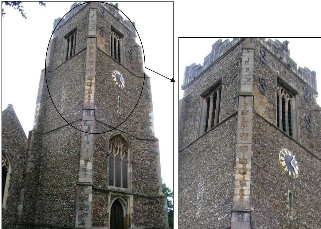
Fig. 3.81: The north west corner of the tower with the upper two stages shown in greater detail in the right image. Note the faint outline of a window opening on the northern face at the second stage and also the different window tracery patterns between the north and west belfry openings.
