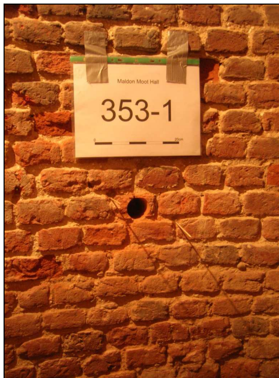
Fig. 3.40: The brickwork surrounding the sampling point at the base of the brick newel staircase in the Moot Hall, Maldon. The scale bar is 20 cm in length.
