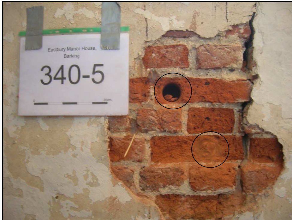
Fig. 3.20: The exposed fragment of brickwork in the western wall of the cupboard in the panelled room. The sampling locations have been circled. The scale bar is 20 cm in length. The image illustrates the aesthetic impact the sampling has on the brickwork since the lower of the two sample core holes in this image has been repaired and allowed to dry over the course of several months.
