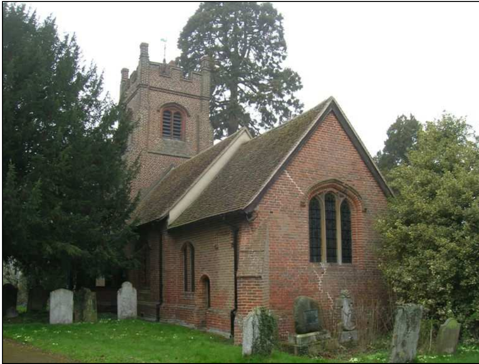
Fig. 2.9: Chignal Smealey church, a rare example of a church built entirely from brick in the early 16 th century.
