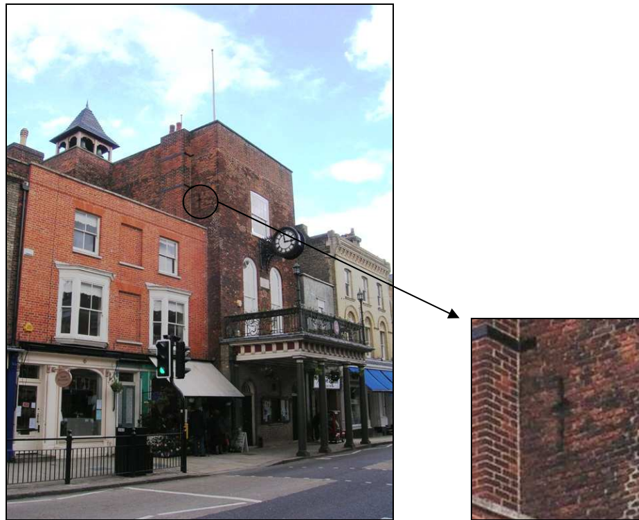
Fig. 3.30: Maldon Moot Hall. The image on the right shows the blocked cruciform arrow loop, a feature more likely intended for ornamentation than serious defence of the tower house.
