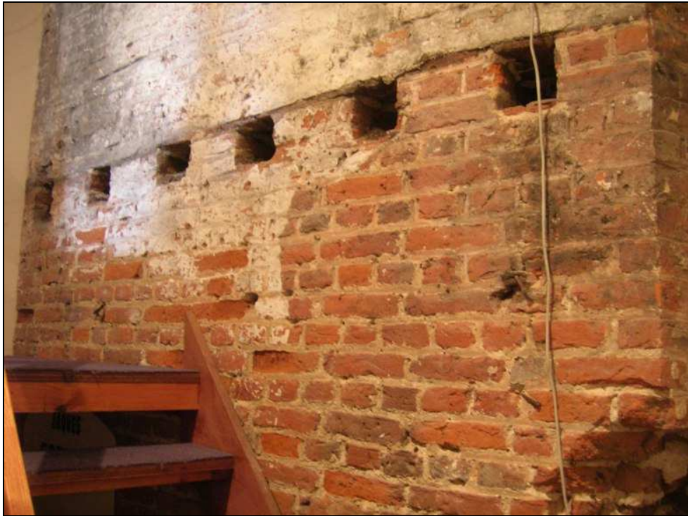
Fig. 3.31: Holes in the wall just above the modern first floor level. This wall extends eastwards from the Moot Hall and into the first floor of the adjacent building. It is thought that the holes may have held corbels to support the roof (see Fig. 3.34).
