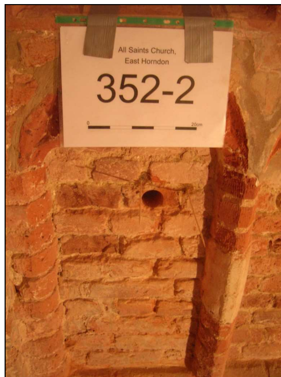
Fig. 3.87: The niche in the eastern wall of Thomas Tyrell's tomb niche. The label is covering the decorative cinquefoil corbelling located at the top of the niche. The irregularities of the bricks in this location contrast the modern replacement material located in other areas of the niche, suggesting this is authentic 'Tudor' type brick. The scale bar is 20 cm in length.
