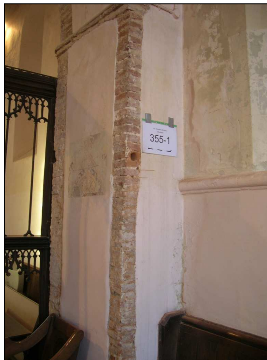
Fig. 3.75: The sampling point on the northern respond of the arch between the tower and the chancel after the core had been removed. The scale bar is 20 cm in length.
