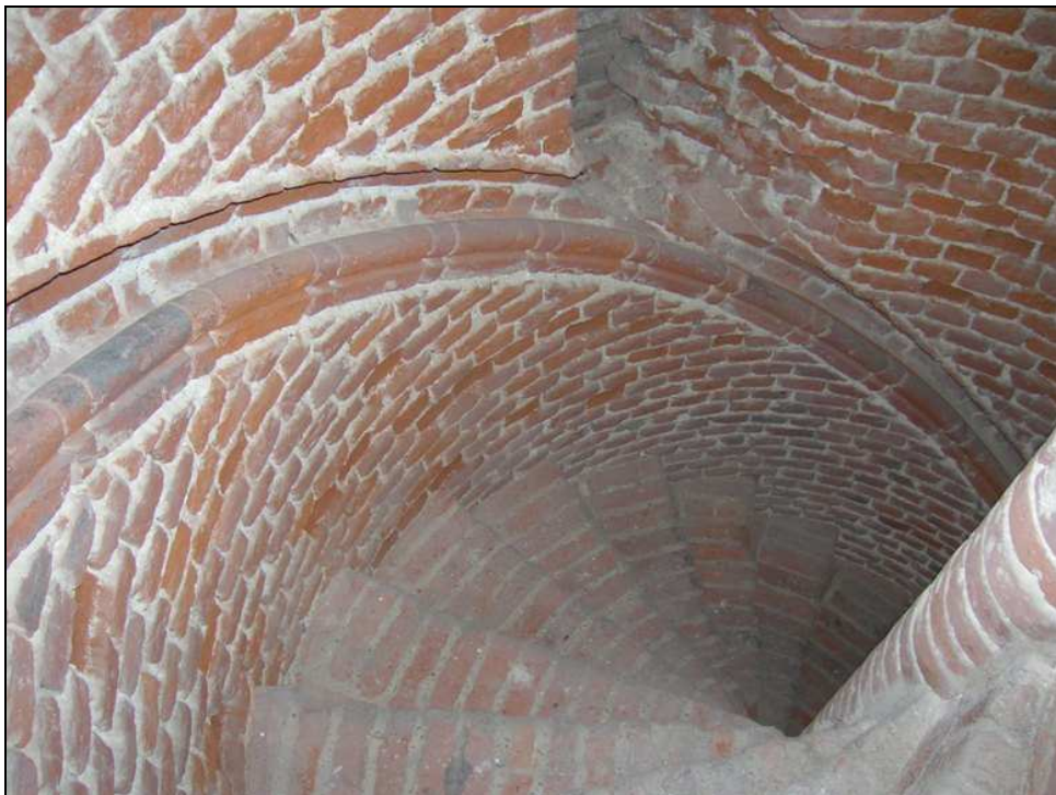
Fig. 3.38: The view down the brick newel staircase, illustrating the header bonded wall, the brick treads, the brick newel post and the alternating stretcher-header pattern of the moulded brick handrail.
