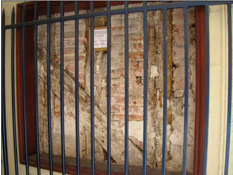
Fig. 3.35: Remains of a timber framed structure with brick nogging infill located to the east of the Moot Hall.
