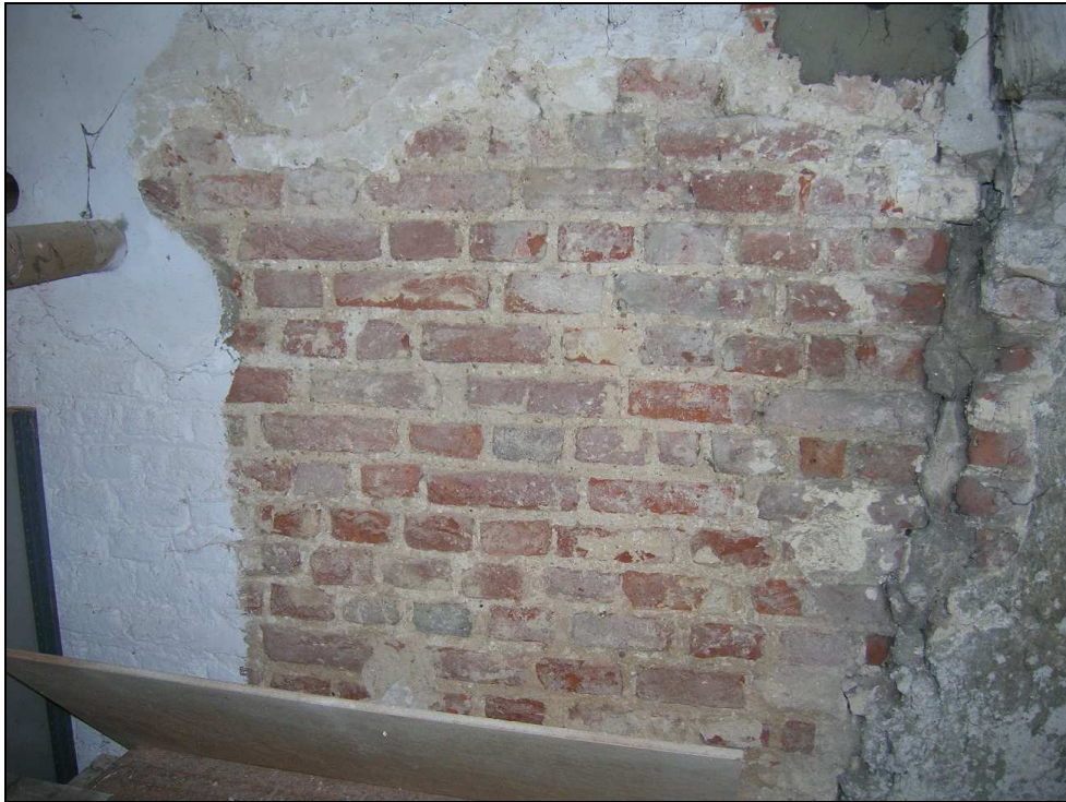
Fig. 5.4: Exposed brickwork in New Hall cellar with an irregular bonding pattern.
