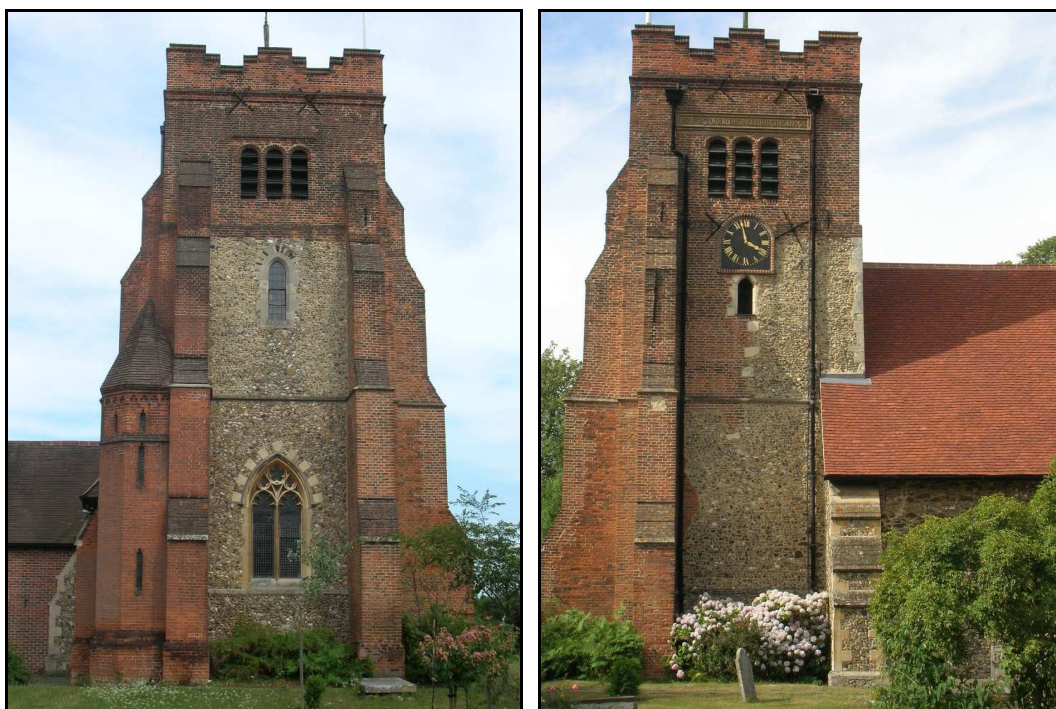
Fig. 3.98: The western tower at Springfield as seen from the west (left image) and the south (right image). Note the extensive use of brick for the third stage and the corner buttressing.
