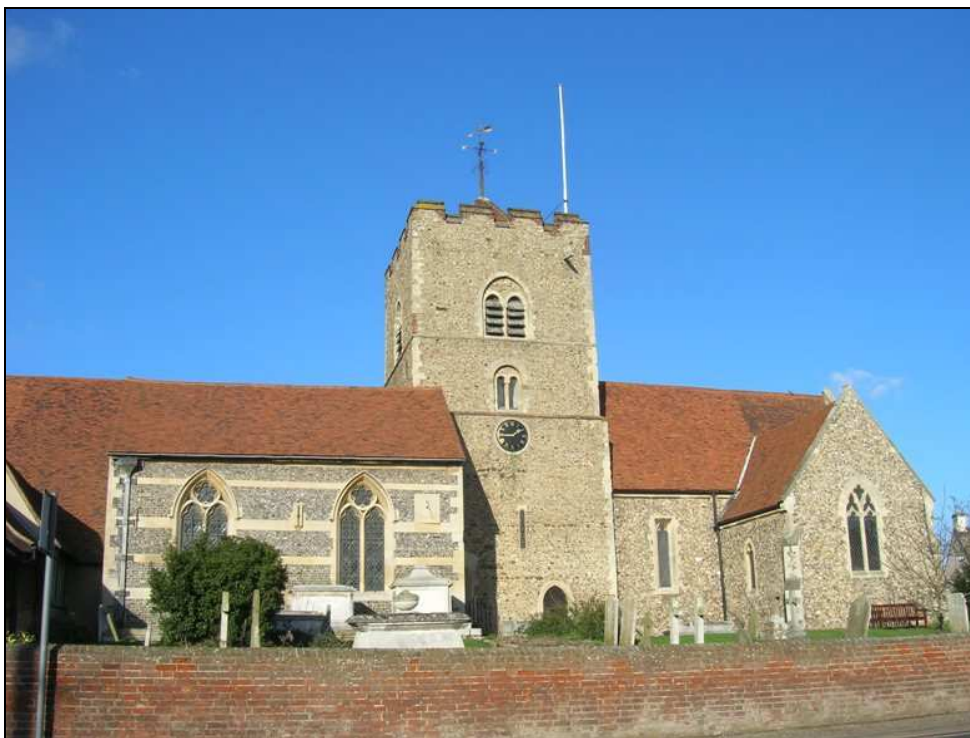
Fig. 3.68: St. Andrew's church, Boreham. Note the unusual layout of the building with the tower in the centre, the chancel to the east (right side in the image) and the aisled nave to the west (left side in the image).
