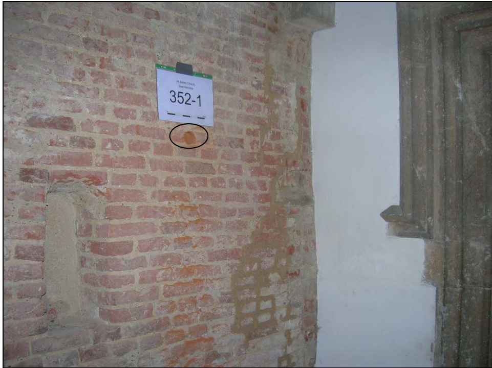
Fig. 3.86: The sample point (circled) of the south porch internal western wall. The scale bar is 20 cm in length. Note the small niche, possibly a stoup, to the left of the image.
