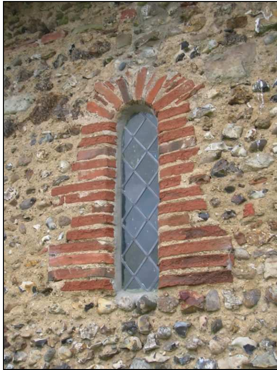
Fig. 3.76: The use of medieval bricks in the Norman window surrounds at Bradwell-juxta-Coggeshall, one of the three main contexts in which medieval bricks are used at Bradwell-juxta-Coggeshall church.
