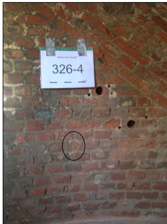
Fig. 3.48: The sampling points at the base of the brick newel stair. Note the change in the bonding pattern in the top right corner of the image. This change signifies the springing of the spiralling barrel vault upon which the lower part of the staircase sits. The scale in the image is 20 cm in length. There are three sampling points, two of which are shown open. The other sampling point is circled. This point was repaired and allowed to dry over the course of several months, illustrating the aesthetic effectiveness of the repair work undertaken.
