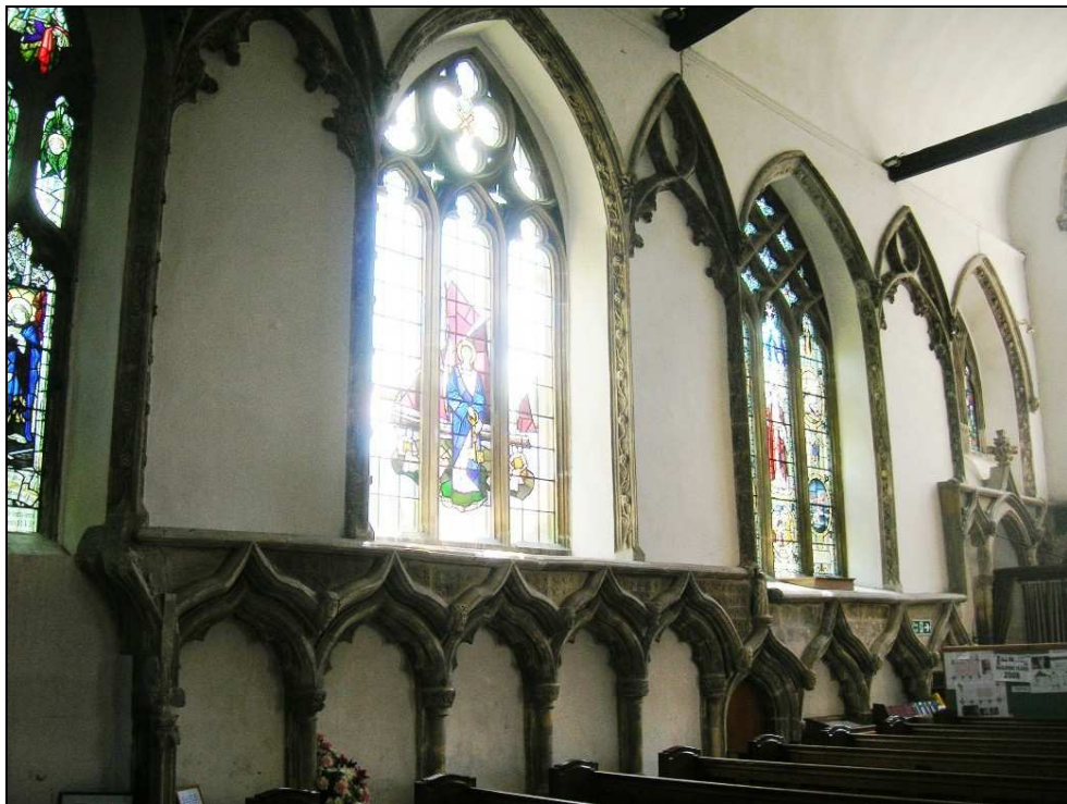
Fig. 3.94: The internal view of the south wall to the south aisle. Note the five niches with ogee moulded heads to the left of the image. On the right of the image there are three further niches at a slightly lower level. At the junction of the two series of niches is the entrance to the sunken chamber.
