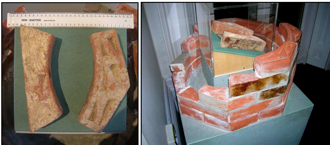
Fig. 2.14: Medieval chimney bricks. The left image shows the two different forms of brick needed to produce a chimney (the left brick is a ‘Type B’ brick whilst the right brick is a ‘Type A’ brick. Note the keying holes in the Type A brick). The image on the right demonstrates how alternating courses of the two types of brick produce a cylindrical shaft with an octagonal exterior.
