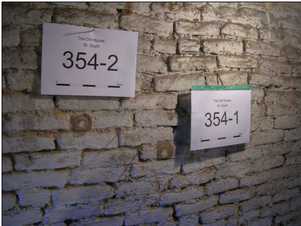
Fig. 3.66: The southern wall of the cellar at ‘The Old House’. The two sampling points had recently been repaired when this image was taken. Both of the scale bars are 20 cm in length. Note that whilst the brickwork of the wall is largely laid in stretcher bonding, there are irregularities. These include occasional header faces in the uneven courses.
