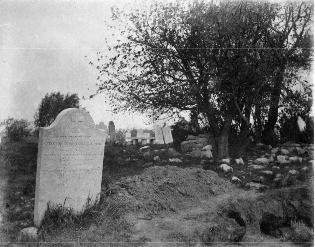
Plate 9 - A photo showing the state of the Upper Burial Ground prior to its conversion to a park. Note the exposed dirt, debris, and leaning tombstones. The grounds would have been very muddy after rain and in spring.
