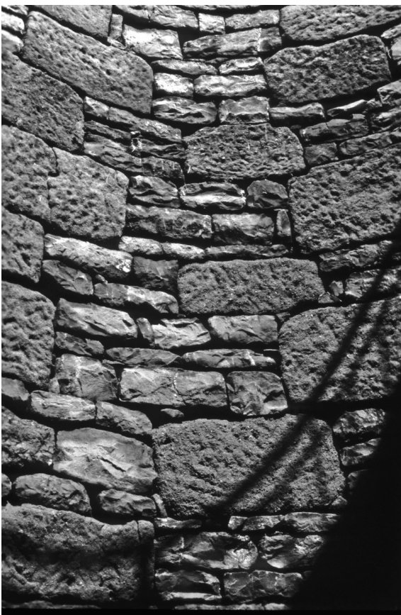
Figure 12. Interior of the so-called “Pozzo sacro”, showing the building technique a scacchiera with the use of sandstone and flysch.
