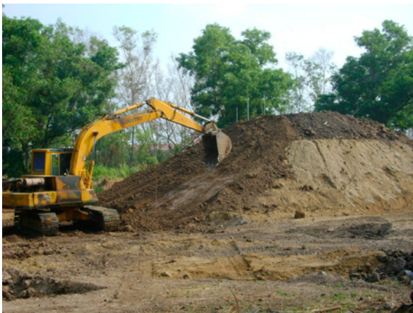
Fig. 7 The construction of embankment slope (1V:1.5H) for monitoring
