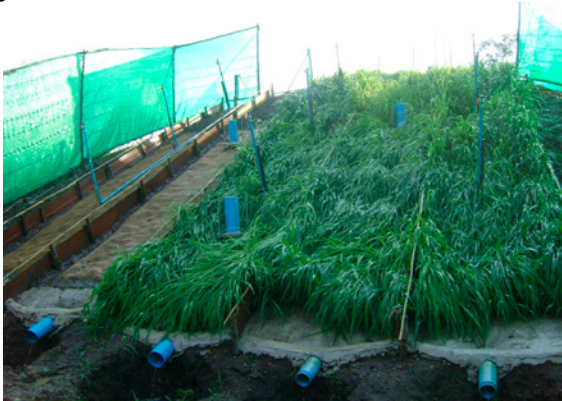
Fig. 11. The embankment at east side
