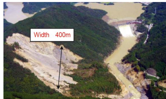
Fig. 3. Large landslide downstream of the Tsukabaru dam.
