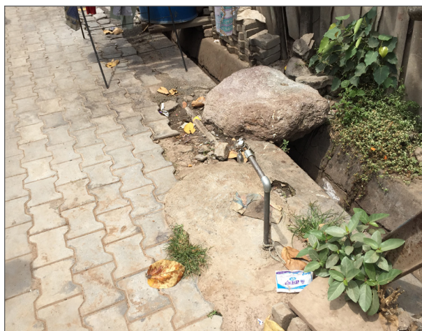
FIGURE 18: OPEN DRAINAGE ALONGSIDE A WATER PIPE NETWORK IN A NOTIFIED SLUM IN PUNE
