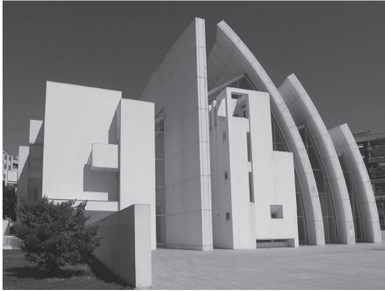
Fig. 4. Church Dives in Misericordia, Rome, Italy designed by architect Richard Meier who choose to build the structure using cement containing a significant percentage of titanium dioxide, 2003 (source: http://files1.structurae.de/ ).
