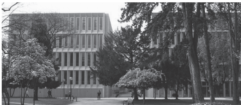
Fig. 3. Cité des Arts et de la Musique, Chambéry, France. This is the first building where mortars containing titanium dioxide were applied, 2000 (source: http://citedesarts.chambery.fr/ ).
