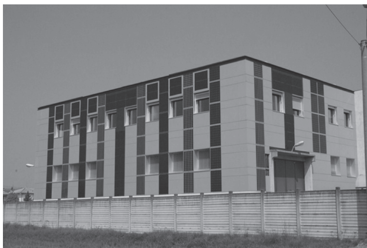
Fig. 5. View of the case study building. Source: www.edilportale.com .
