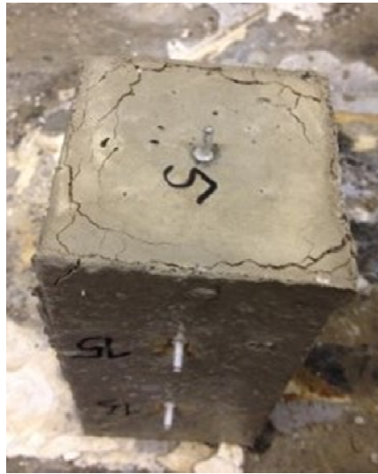
Figure 4 – Cracks pattern on a concrete specimen after 400 days of immersion in a 10% Na 2 SO 4 solution
