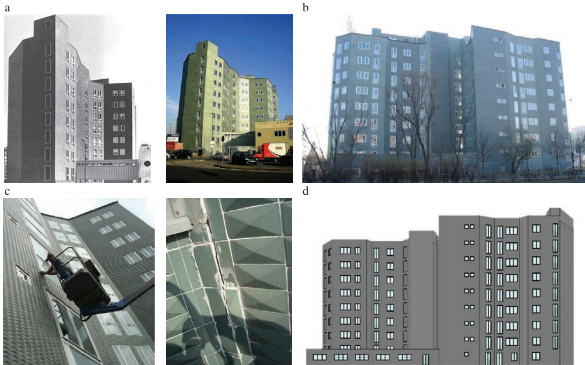
Fig. 3. Historical picture of the Palazzo Savoia Assicurazioni e Riassicurazioni office building (a) and today view; the building had a strong need of refurbishment (c) and the analysis has been base on a BIM model (d) to compute energy needs and quantities.
