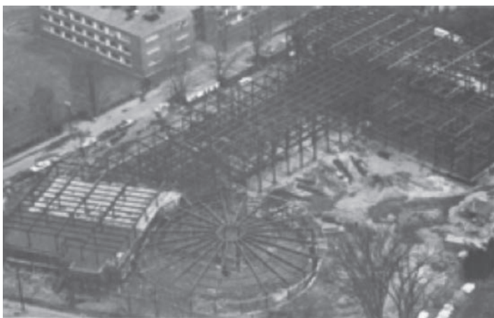
Fig. 8. “G roundbreak and Construction,” The Campus Comment , February 26, 1969.
