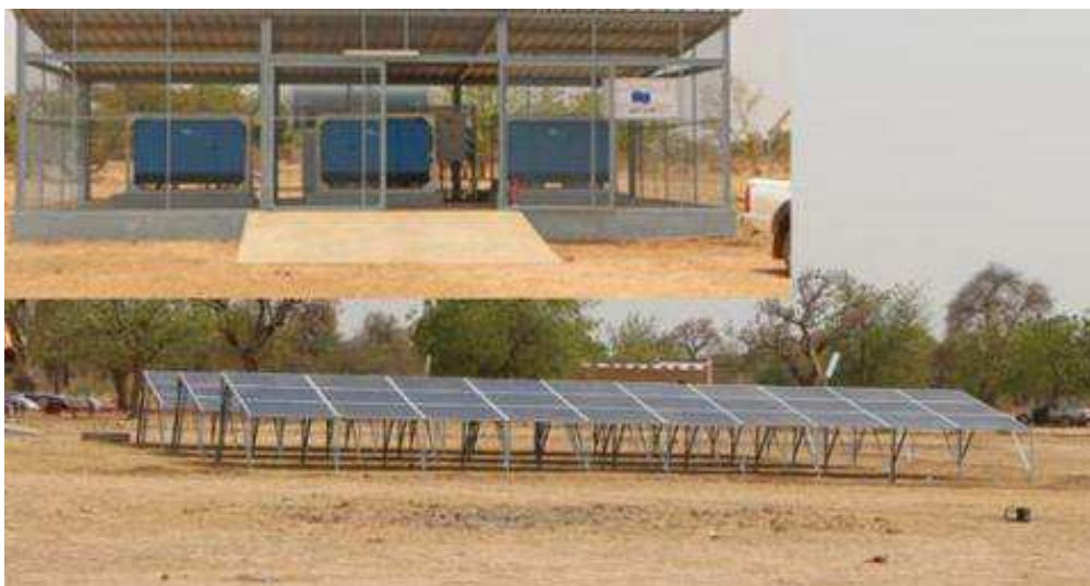
Figure 9. Hybrid PV system in Bilgo (30KW p /77KVA).
