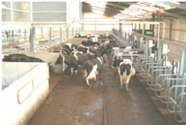
Cubicle house with gate dividing the concrete (near) and rubber flooring (far) areas
