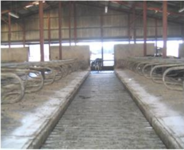
Cubicle house showing passageway covered with slat mats (MODIFIED treatment)
