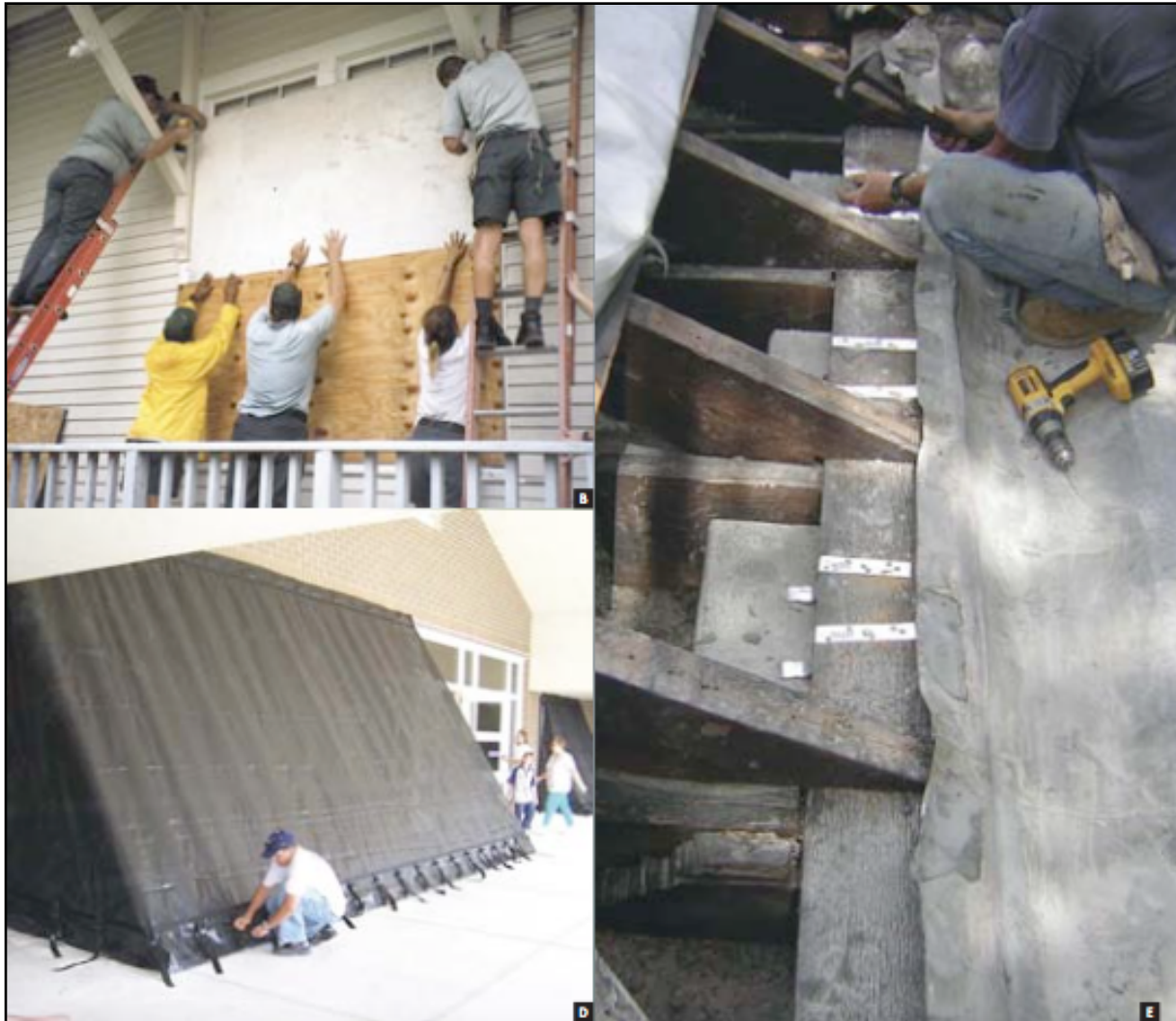
FIGURE 8: Storm Preparation Measures in Florida. Clockwise from top left: Koreshan windows' protection added (plywood held with screws). Top plates being secured to wall plates and pillars. Temporary wind abatements added to protect foyer doors and windows. (1000 Friends, 2008:8).
