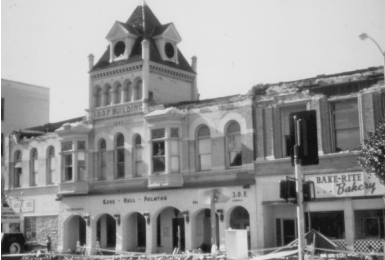
FIGURE 3: A Case of Retribution. The Oddfellows' Fraternal Hall, Watsonville, CA, was damaged during the 1989 Loma Prieta earthquake, the falling parapet masonry killing a pedestrian. Although repairable, the building was quickly demolished a few days after the disaster. The tower had been, indeed, a wood frame construction with metal covering and did not fail during the earthquake event. (Photo: Steade Craigo 1989). (Spenneman and Look, 1998:178).
