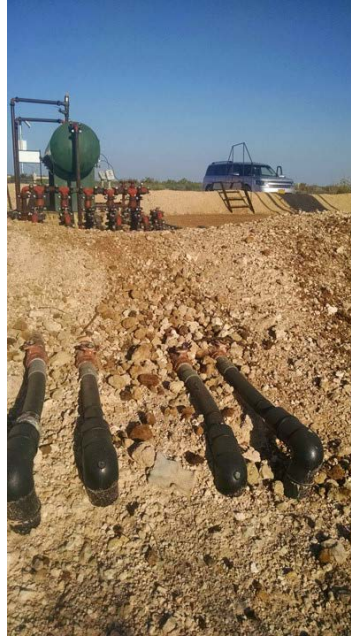
Fig. 1-12. Gathering pipes lead to the Battery (photograph taken by author).
