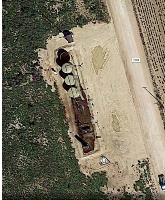
Fig. 5-1. Hatchett deployment site with weather station visible
