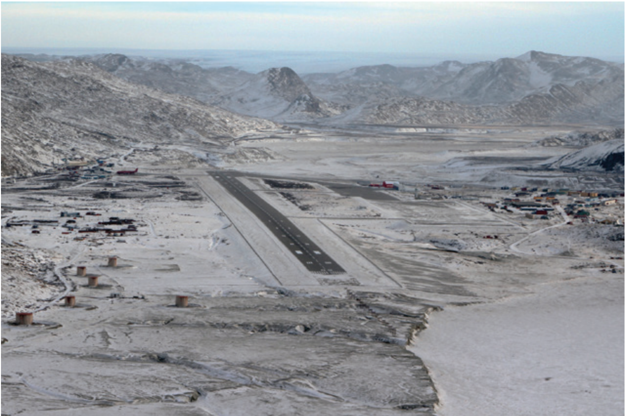
Figure 10.12 The Kangerlussuaq airport and its supporting settlement are located on the river terrace of a glaciomarine delta, in close proximity to the Greenland Ice Sheet (visible in the background) (photo by Thomas Ingeman-Nielsen).
