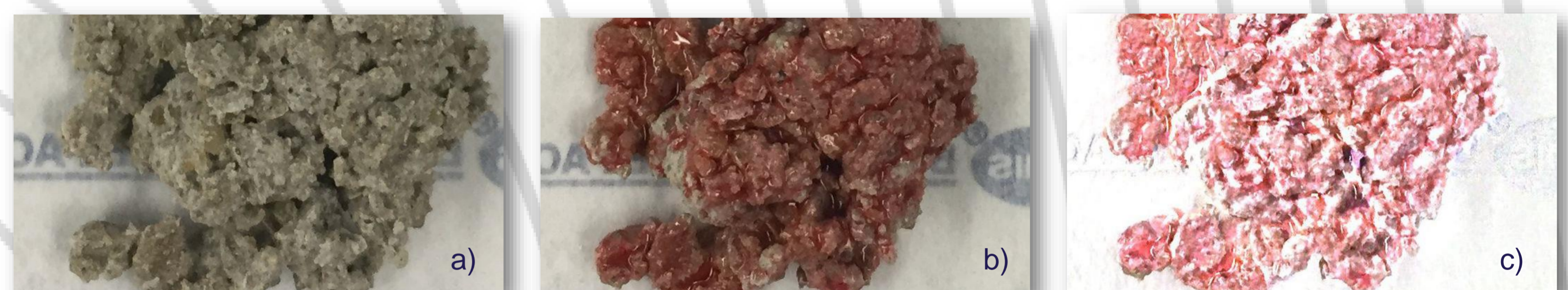
Figure 3. Images of corroding concrete before (a) and after (b) application of the pH indicator. Colour enhancement by "divide filtering"; i.e., dividing the intensity of each color channel (R,G,B) in every pixels (c).
