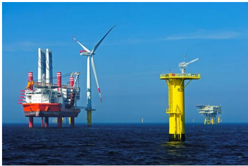
Installation of a wind turbine on a monopile ( www.4coffshore.com ).
