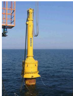
Up-close of installation of offshore piles ( www.4coffshore.com ).
