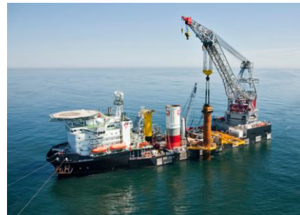
A vessel used for installation of piles for offshore wind turbines ( www.cape-holland.com ).
