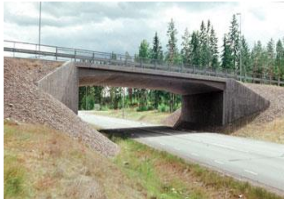
Figure 1. A concrete slab frame bridge [18]
