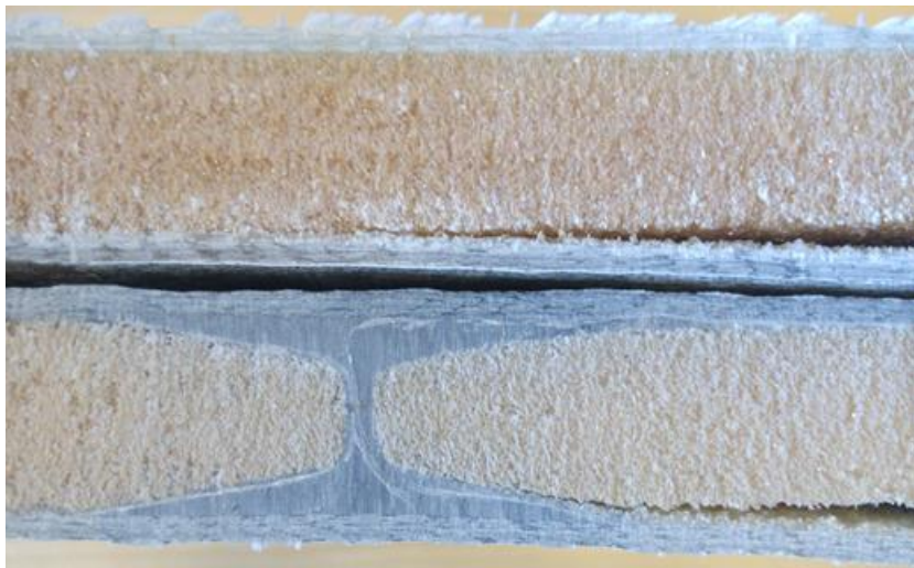
Figure 11. Post mortem sections of sandwich panel specimens PLT2 (above – no peel stopper) and PLP2 (below - with embedded peel stopper).
