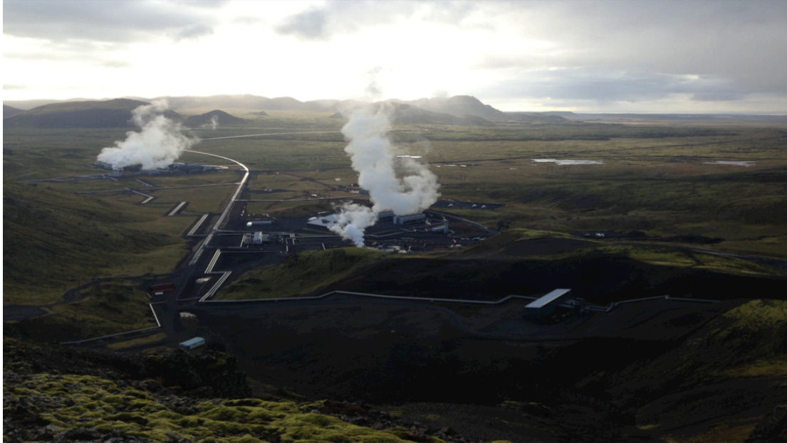
Figure 3: Hellisheiði Geothermal Power Plant, Hengill in late September.
