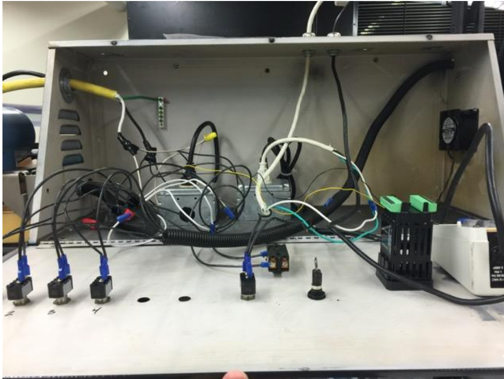
Figure 20. Before photo of the inside of the enclosure.
