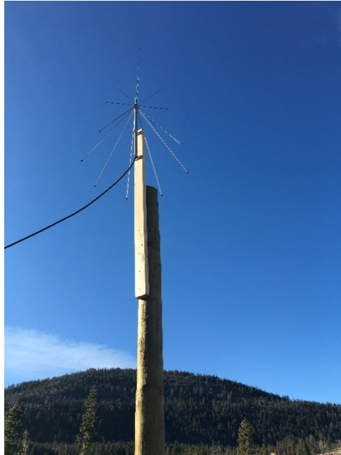
Figure 19: Discone Antenna at Moose Lake Road Location
