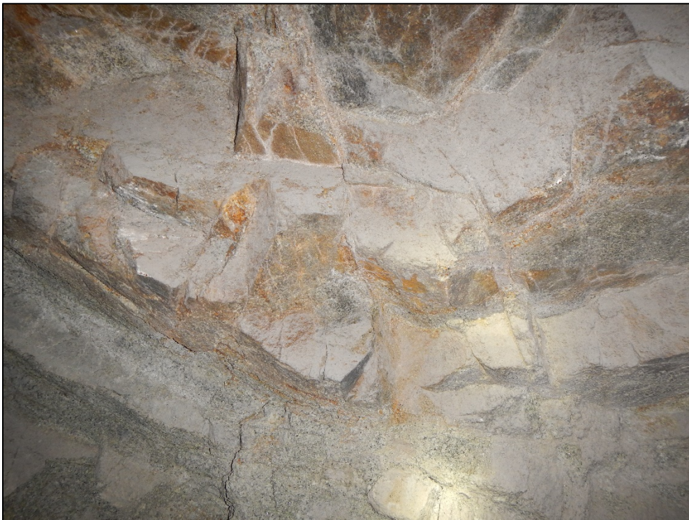
Figure 21: Weathering Grade II observed at UMEC.
