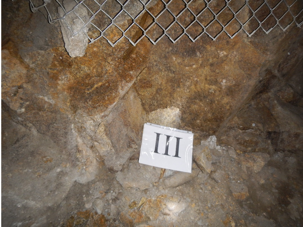
Figure 22: Weathering Grade III observed at UMEC.
