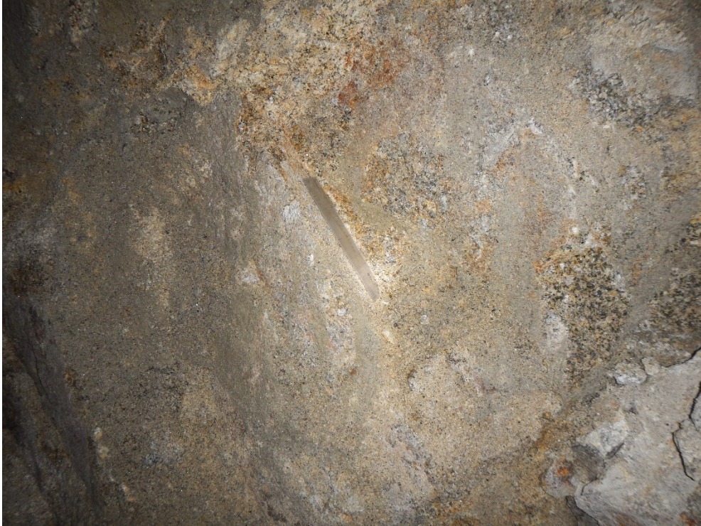
Figure 24: Weathering Grade V observed at UMEC.
