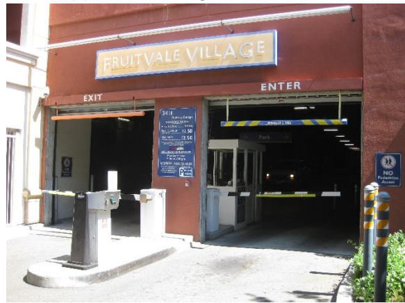
(f) Shared parking garage entrance for 3411
