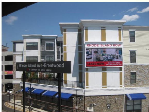
a) North building as seen from Metro platform
