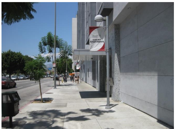
(h) Vermont Avenue residential entrance
