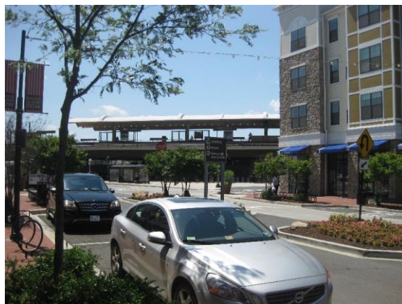
b) Metro platform and bus bays
