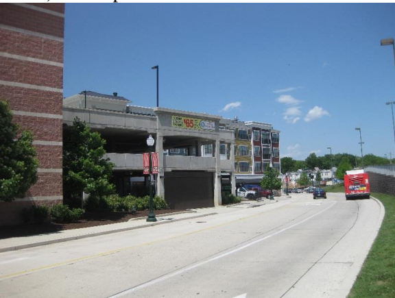
g) South parking garage
