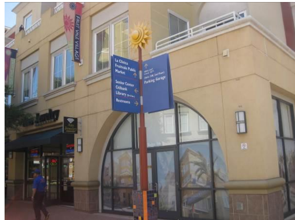
(b) Apartments above shops
