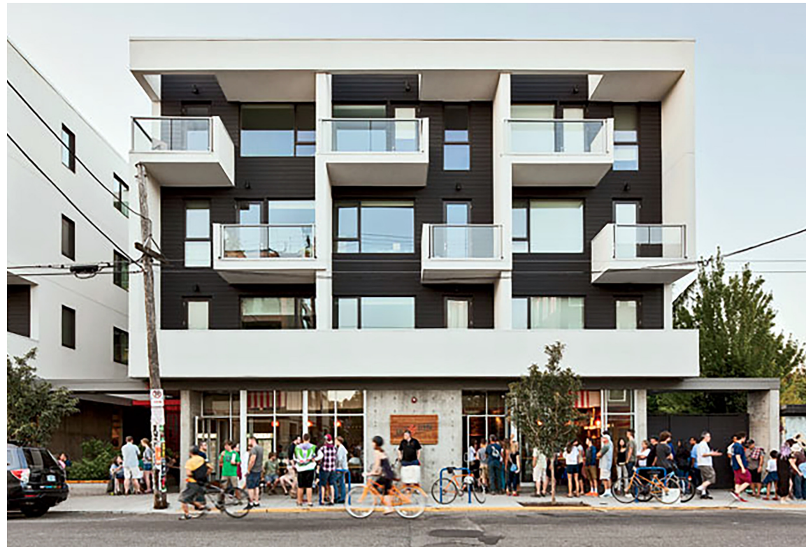
Above: Enhanced Pedestrian Frontage
