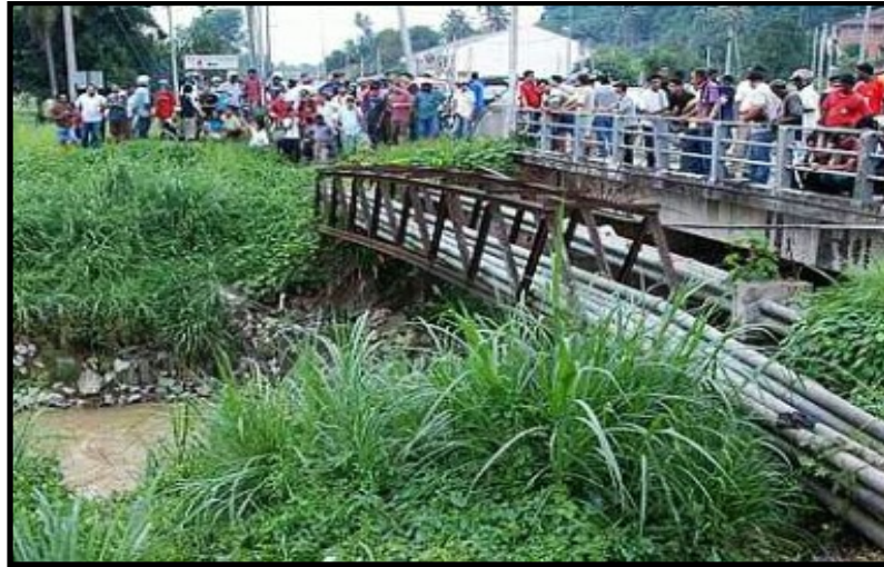
Fig. 9.1: Pinji River on the day the bomb was found (source: The Star 17 June 2008)
