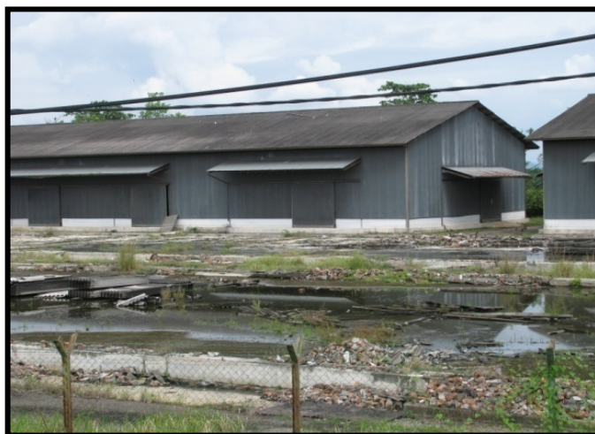
Fig. 7.2: LPN building in Bagan Serai (source: author)
