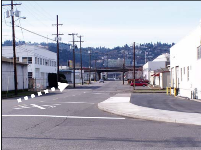
Looking down SE Division Place from the NE corner of SE 8th — a large turning radius for trucks increases the crossing distance to 64 feet. Pedestrians are encouraged to cross SE 8th on the south side.
