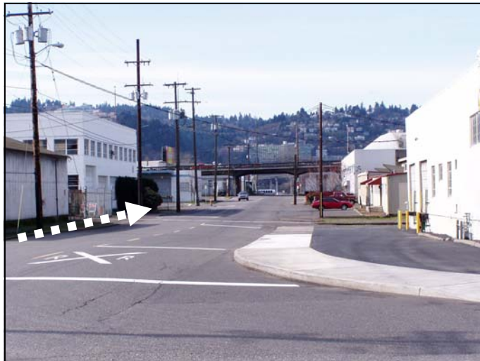
Looking down SE Division Place from the NE corner of SE 8th — a large turning radius for trucks increases the crossing distance to 64 feet. Pedestrians are encouraged to cross SE 8th on the south side.
